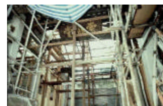
Temporary structural supporting and working platform falsework
