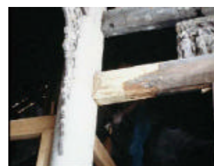
Replacement of deteriorated timber structure in Kun Ting Study Hall
