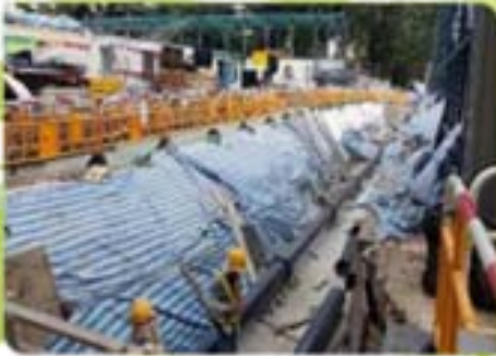
Cover on Excavated Surface 3
