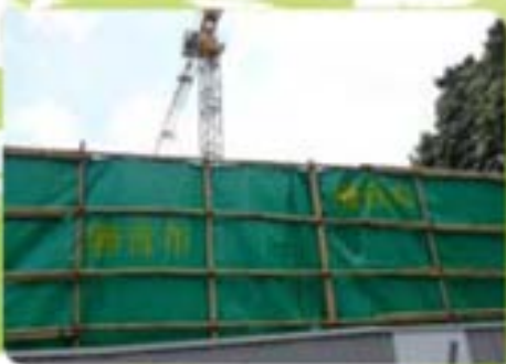
Sound Barriers around Construction Site 2
