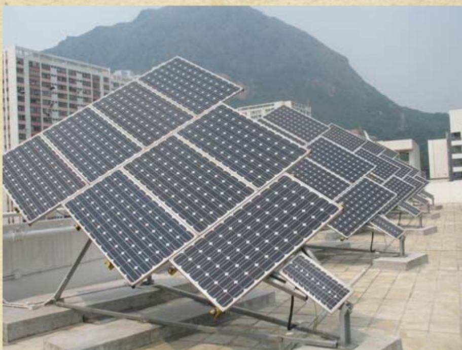
PV Panels with Sun Tracking System
