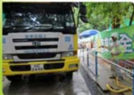
Treated Water Recycled for Wheel Wash 2
