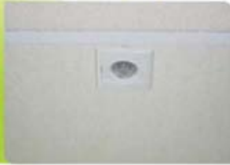
Motion Sensor for Office Lighting 4
