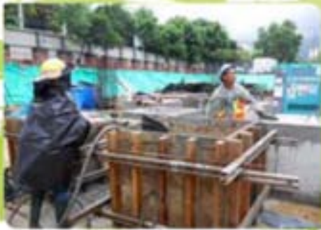
Use of Surplus Concrete for Building Block 5
