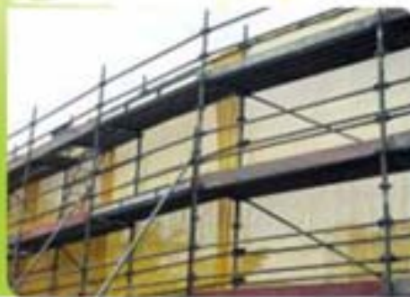
Apply Metal Scaffold instead of Bamboo Scaffold 6
