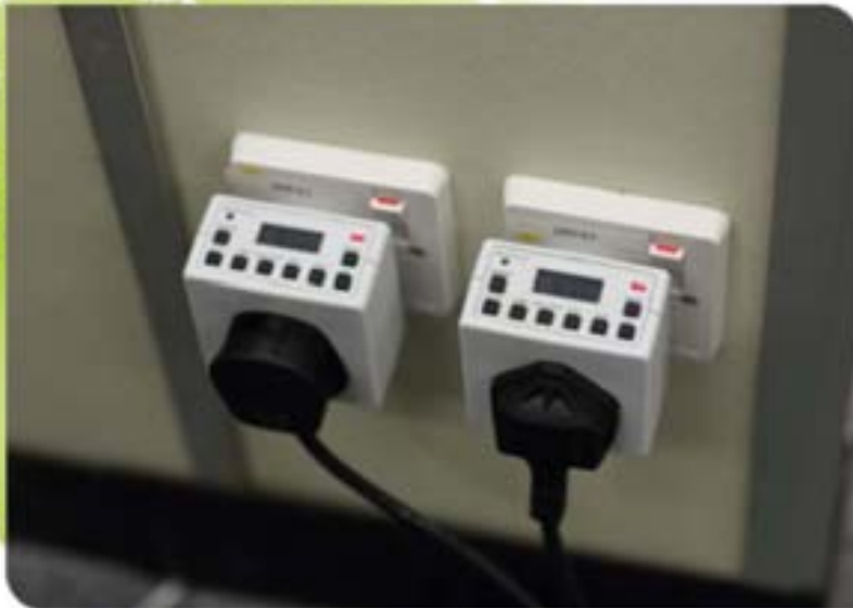
Timers Switches for Office Equipment
