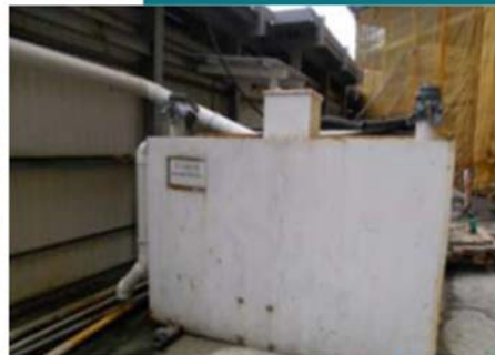
Usage of rainwater recycling for toilet flushing; plant watering and other uses
