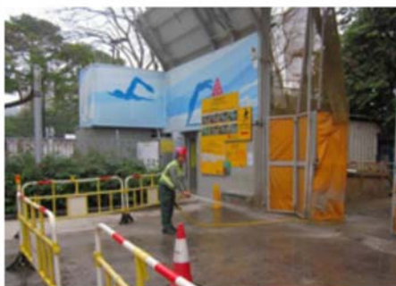
Adopt spray sprinkler system at site entrance
