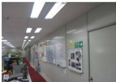
Use of highly energy efficient T-5 lamps and LED lights and provision of "Zoning" for light switches
