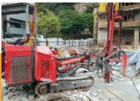
Combination of drilling machine and breakers
