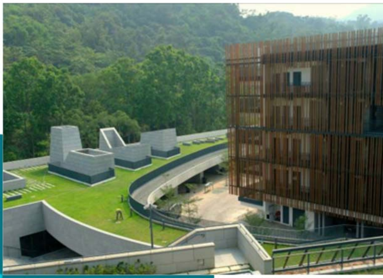
Timber screen shielding of the niches
