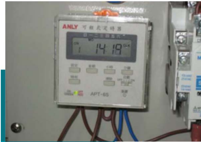
Installation of timer switch for controlling the power supply of non-essential power sockets
