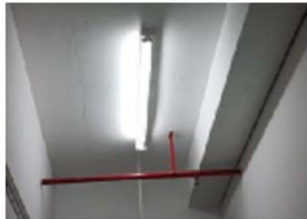
LED lamp with motion sensor installed
