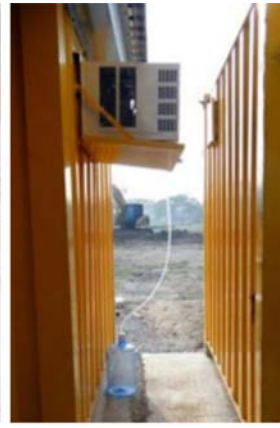
Collect water from air conditioner for reuse
