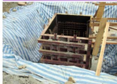
Make use of reusable steel moulds to replace timber formwork
