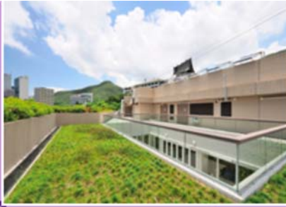
Green roof installation
