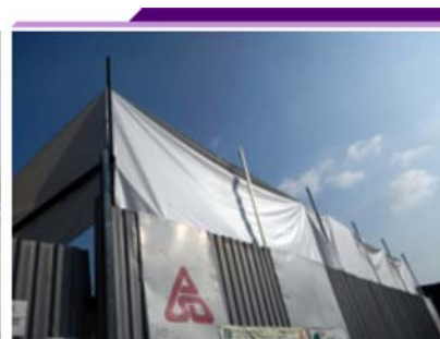
Erection of Dust Screen
