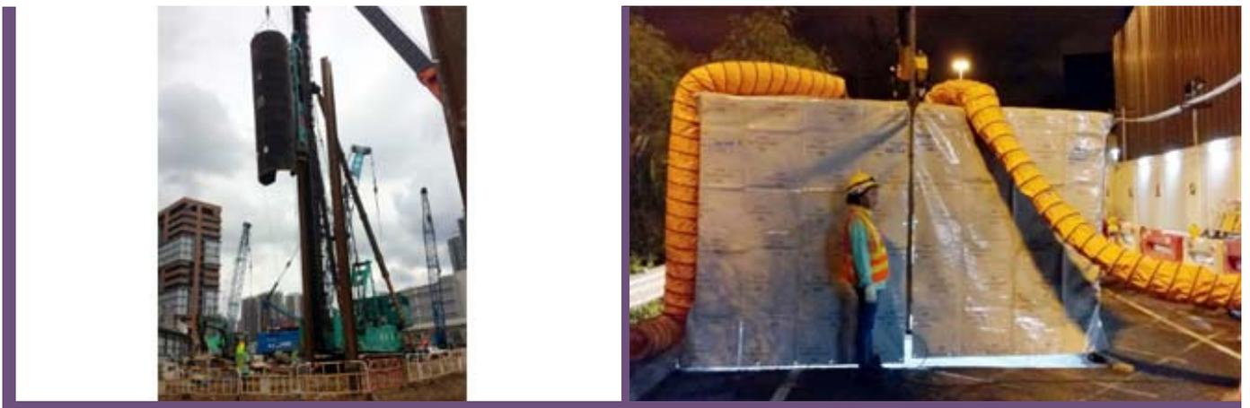
Noise Enclosures for Percussive Piling (Left) and Night Works (Right)<sup>2</sup>
