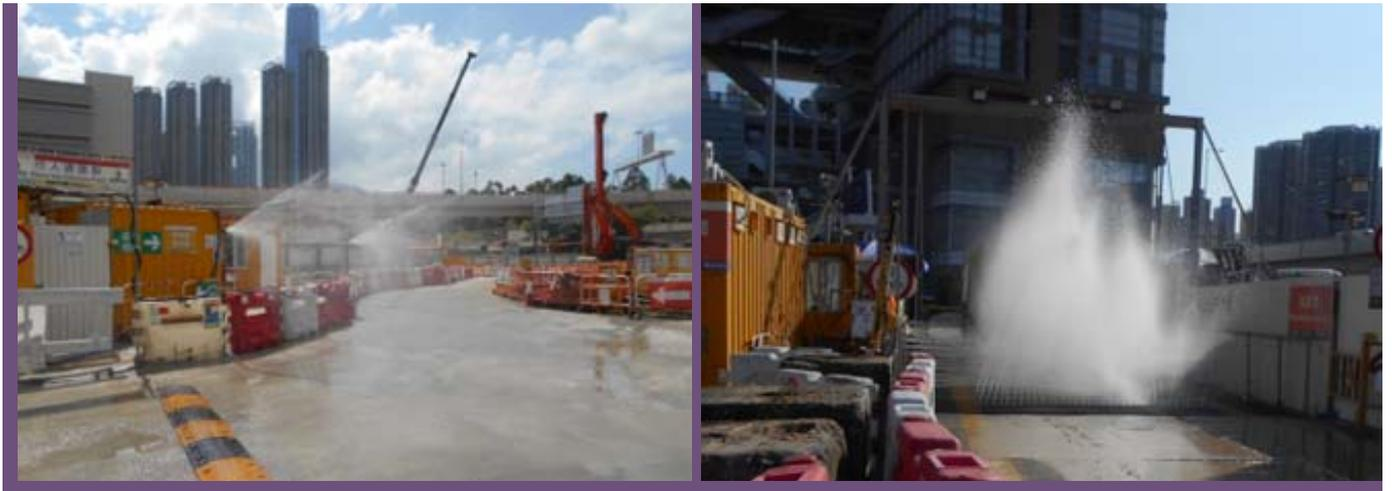
Automatic Water Spraying (Left) and Wheel Washing System with Recycled Water (Right)<sup>2</sup>
