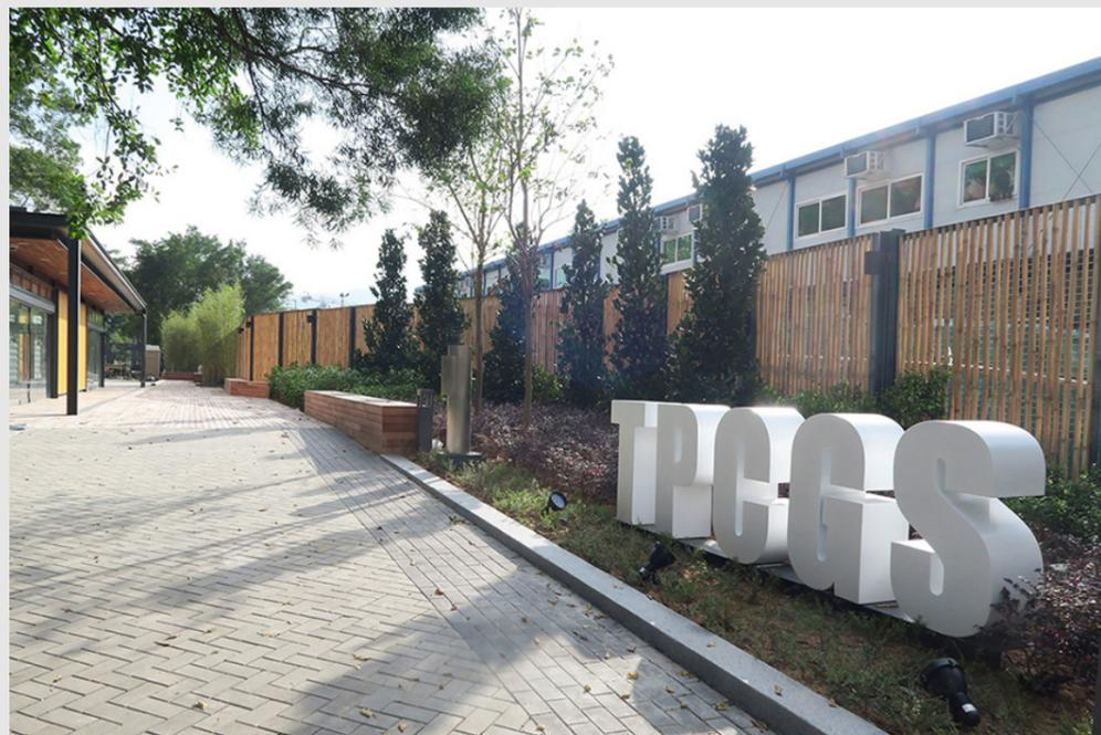
A fence made from reused bamboo
