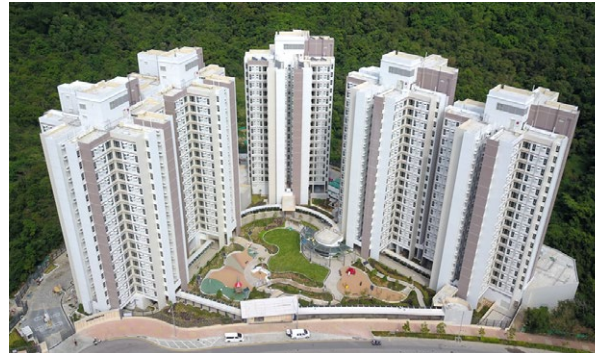
FIRE SERVICES DEPARTMENT PAK SHING KOK MARRIED QUARTERS
