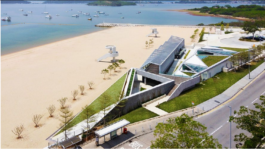
The terracing building improves the connectivity between the access road and the beach
