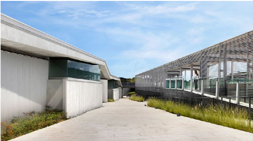
Bamboo-moulded and glass fiber reinforced cement panels as external walls
