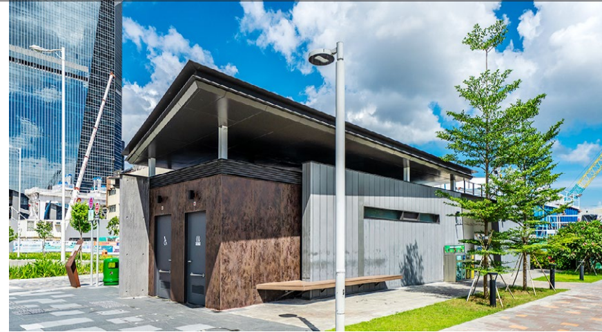
Service block with elderly-friendly toilets and baby care room
