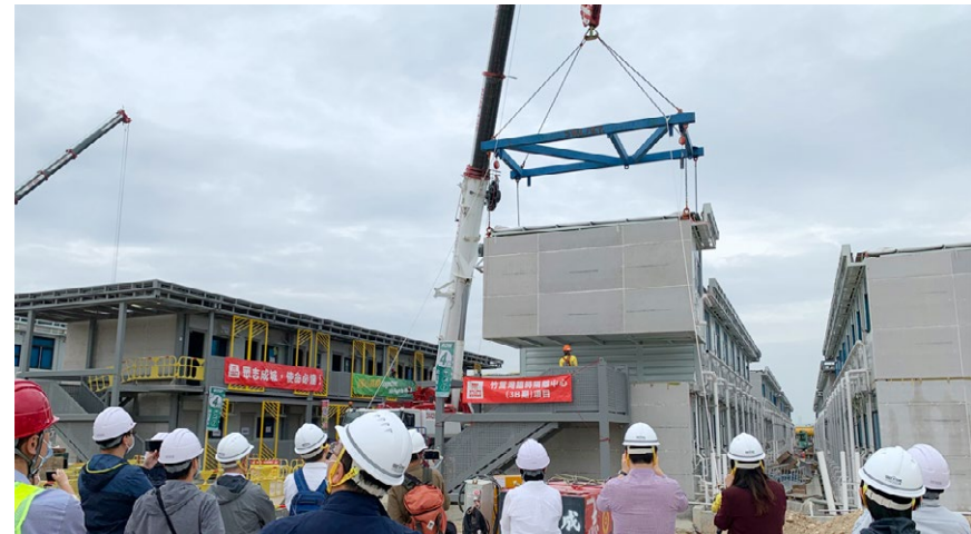
On-site installation of MiC units
