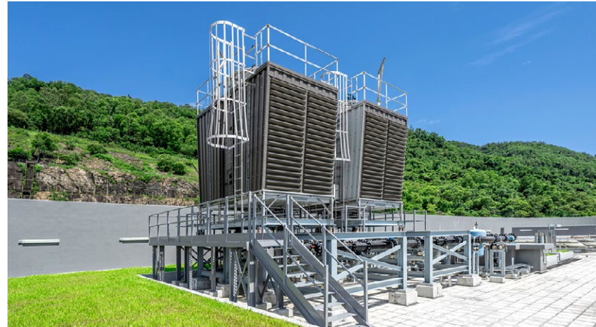
Modular cooling tower and condensing water pipework system
