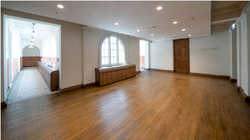
Restored timber floor to retain building character and reduce construction wastes
