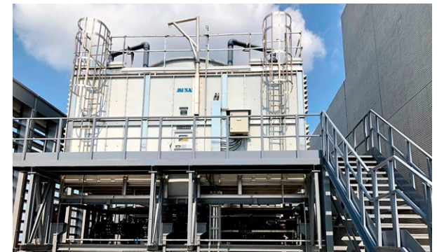
Modular cooling tower & condensing water pipework system
