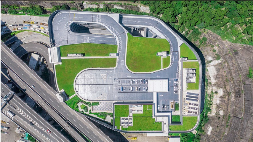
Green roof for heat transfer reduction
