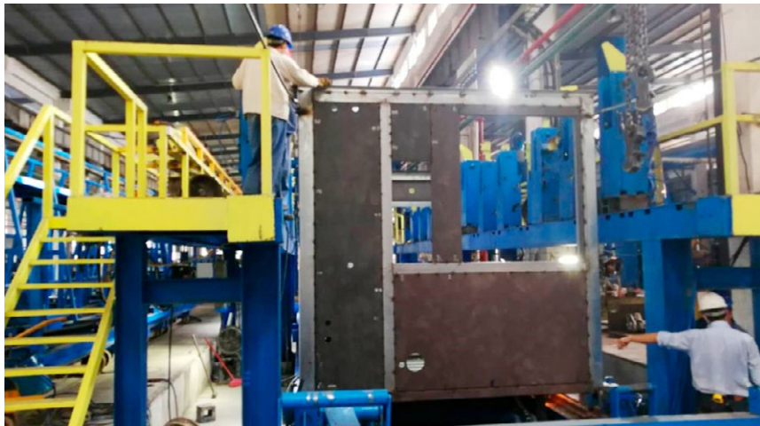
Quarantine units standardised and adopted MiC for off-site fabrication
