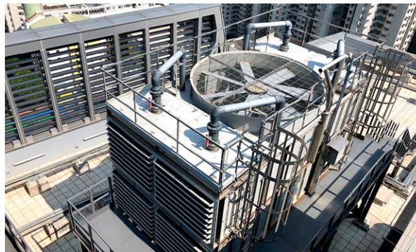
Modular cooling tower & condensing water pipework system
