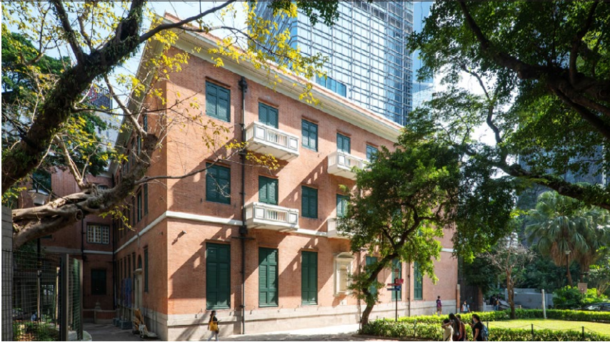
Restored external timber shutters which serve as effective sun shading device since 1919
