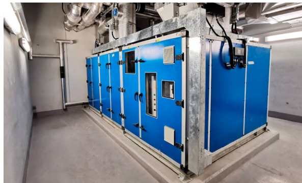
Integrated Air Handling Unit
