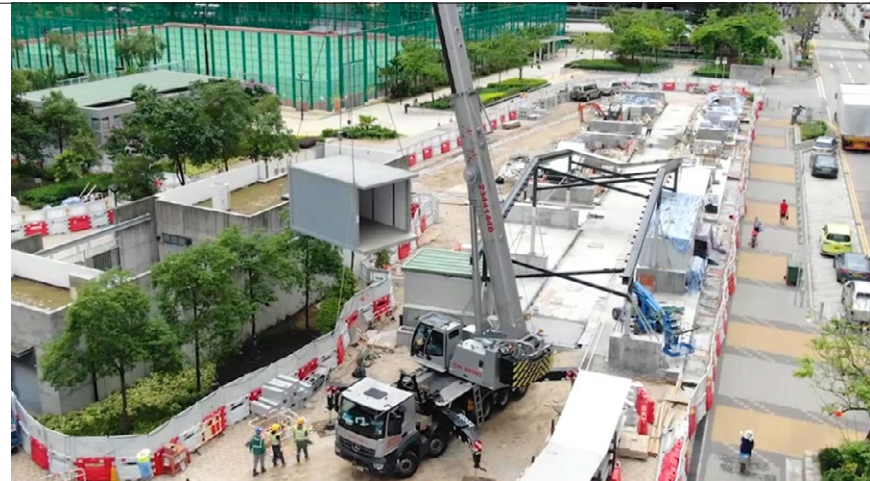
Modules of the MiC containers for market stalls were manufactured off-site and transported to site for assembly
