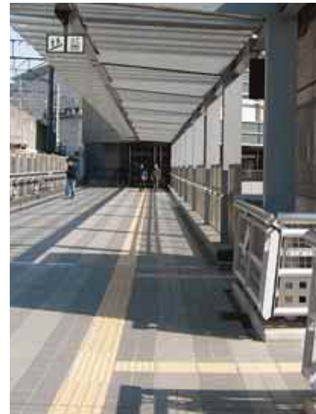
3.1.4.1a Drainage channels positioned along edge of the walkway, away from tactile guide path
