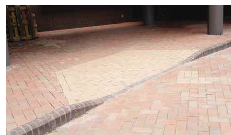
3.1.6.1f Dropped kerb having colour contrast with the adjacent pavement
