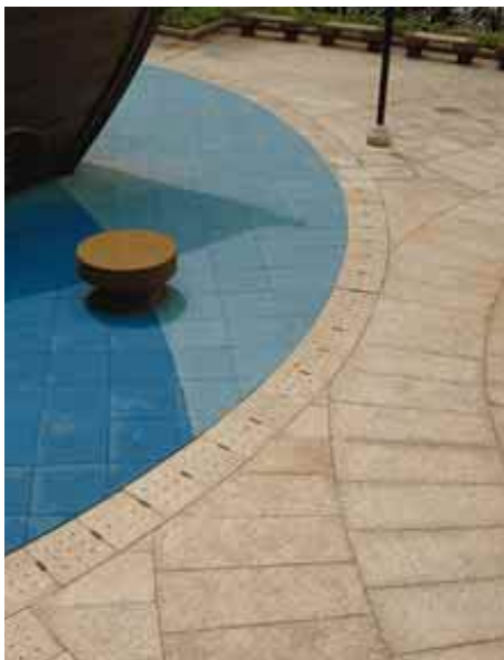
3.1.4.2a Channel covers flush with adjacent floor surfaces with slots less than 13mm wide
