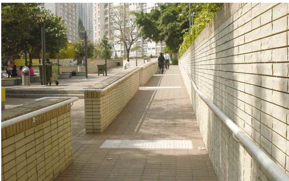
3.1.6.1e Ramp with tactile warning strips, railings on both sides, and colour contrast between the ramp surface and the surrounding walls
