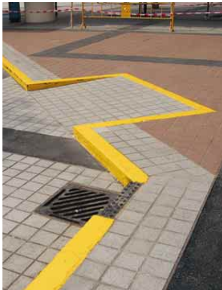
3.1.3.3a Painted warning with colour contrast to adjacent floor finishes at road kerb
