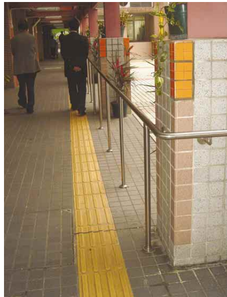
3.1.2.3e Tactile guide path together with handrail provided along access route
