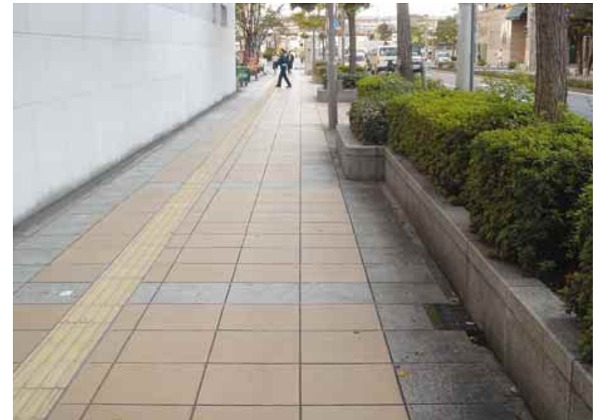
3.1.1b Clear access route free of obstructions and provided with tactile guide path
