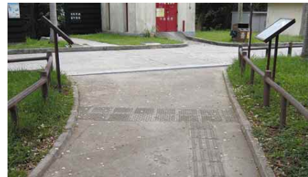
3.1.2.3a Tactile guide path leading to a directory at the park entrance
