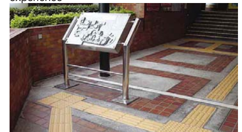
3.1.5.4a Three-dimensional tactile directory led by tactile guide path and audio signals
