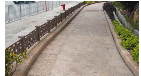
3.1.2.3c Levelled floor surface with kerbs along the pathway to define the access route
