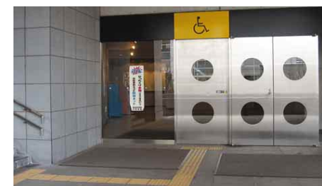
3.1.6.1i Accessible building entrance clearly identified by the international symbol of accessibility
