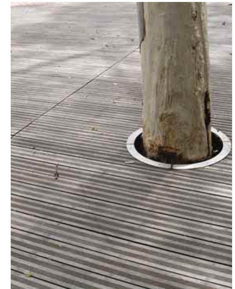
3.1.4.4b Raised flooring with thin slots perpendicular to the travel path to allow surface water to drain underneath
