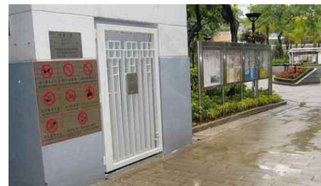
3.1.2.4b Entrance gate recessed into the wall at park entrance providing clear and unobstructed access
