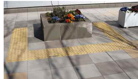
3.1.2.4a Tactile warning strips around planter along the access route
