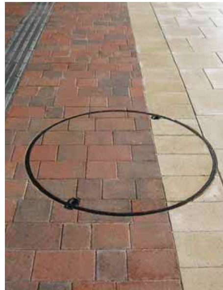
3.1.3.1c Manhole covers levelled with the floor surface
