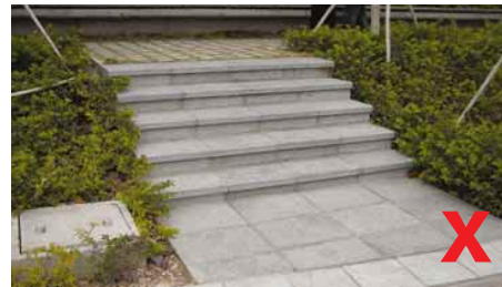
3.1.6.1b Adequate railings and nosing with colour contrast should be provided at stairs and steps
