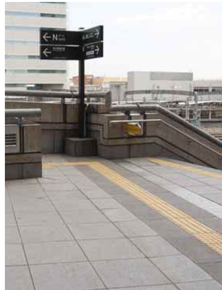
3.1.2.2b Change in levels clearly identified with tactile warning strips
