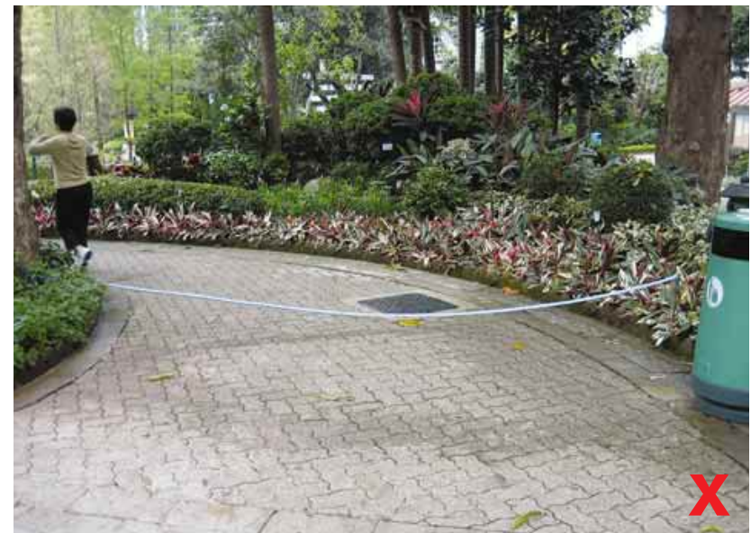
3.10.1b Travel path should be diverted when maintenance work is being carried out
