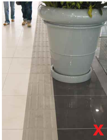
3.10.1a Obstruction to tactile guide path
