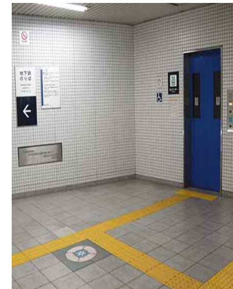
3.2.3.2e Way finding information at change in levels to lead users to their onward destination
