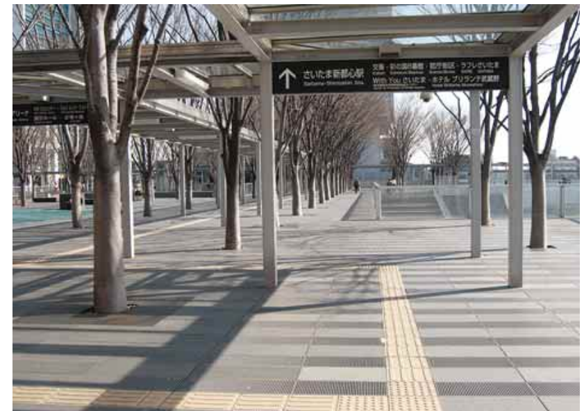
3.2.3.4a Provision of tactile guide path in open space leading to various buildings
