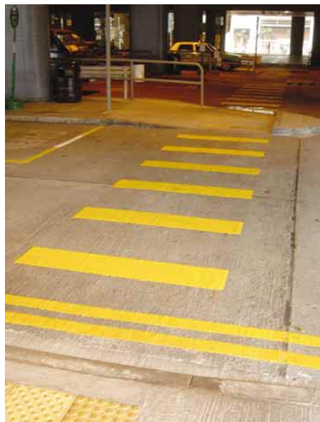
3.2.3.3d Dropped kerbs and tactile warning strips at public transport interchange
