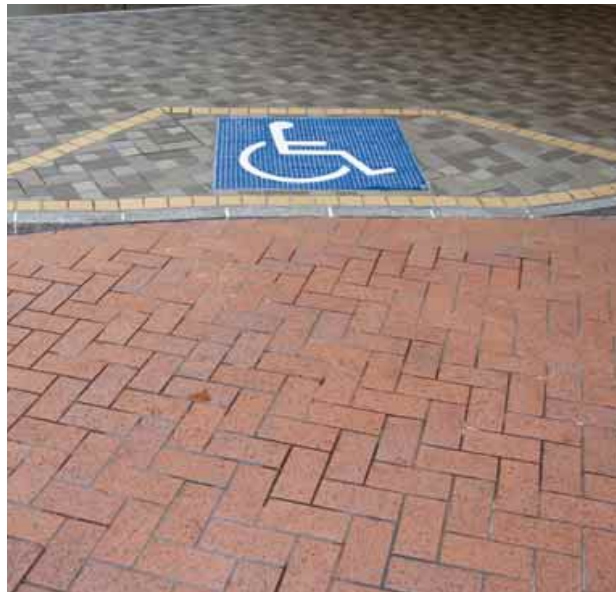
3.2.3.3b Dropped kerb identified with the international symbol for accessibility at a drop-off area
