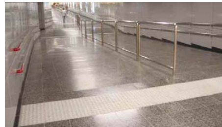
3.2.3.1c Handrails as directional cues to aid users to continue along their travel path at a spatial transition point
