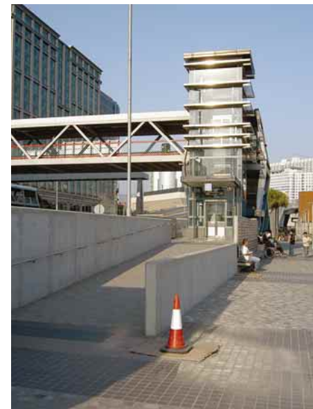
3.2.3.2d Accessible lift at link bridge to facilitate vertical movement
