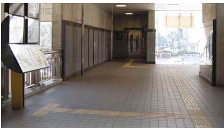
3.2.3.1b Tactile guide path leading from external area to an accessible directory and other destinations
