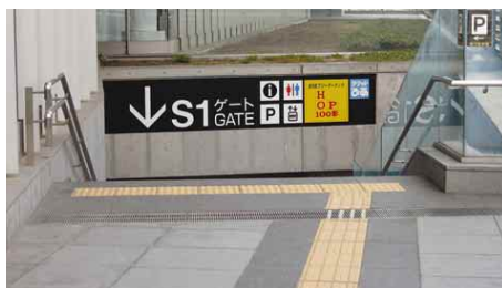
3.2.3.2b Access to a subway led by tactile guide path
