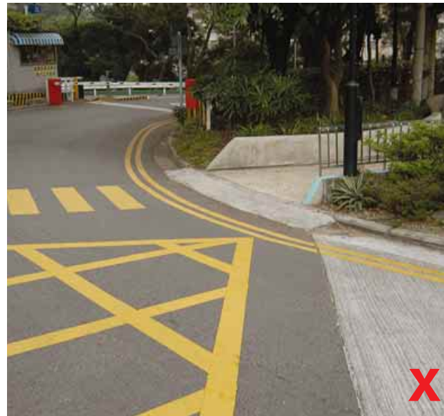
3.2.2a Provision of sloped surface added as afterthought
