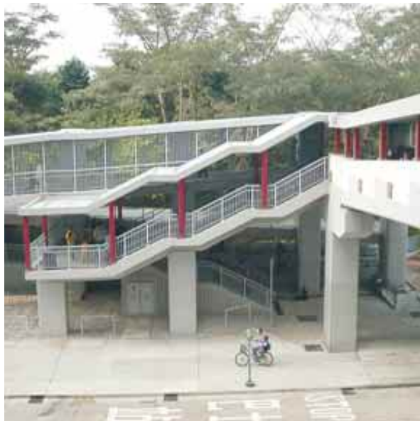
3.2.1a The elevated walkway is commonly used in Hong Kong to connect buildings, facilities and external spaces
