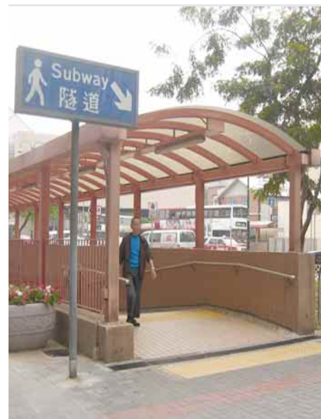
3.2.3.2c Signage and tactile warning strips to indicate entrance to a subway
