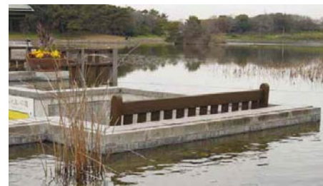
3.3.7.1k Water surface is at a reachable range at this seating pocket, which is also provided with a wheelchair space
