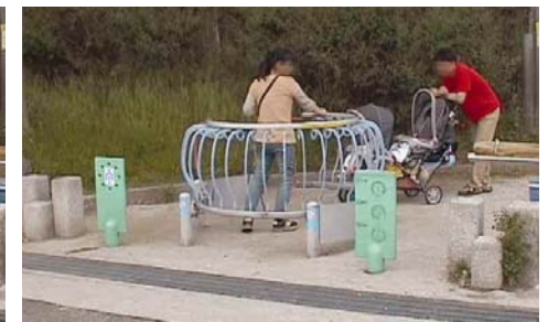
3.3.7.1s Accessible turnstile that controls unauthorized vehicular access
