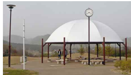
3.3.2.2b Shelters should be centrally located along the access path and the size should cater to the anticipated user rate
