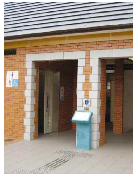
3.3.7.1r Toilet block located at the main entrance
