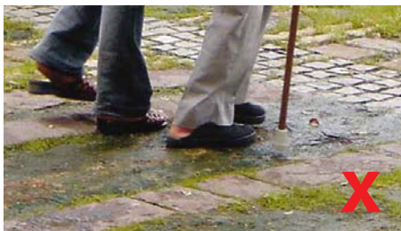
3.3.6.2g Poorly drained lawns are hazardous
