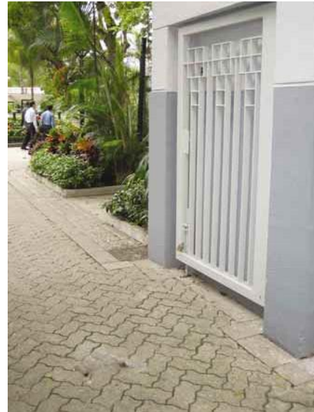
3.4.1.2 a Gate recessed into the wall in open position
