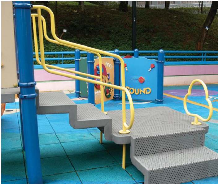
3.4.2.4c Low-level deck with grip bars at different heights facilitates all users to get on/off the play equipment
