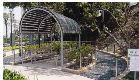
3.4.3.1 b Handrail, warning sign and rain shelter with seats provided near a pebble walk
