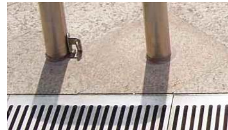
3.4.1.2f Locking device securing a guardrail post
