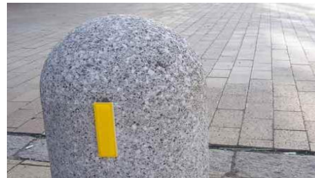
3.4.1.3c Bollard with reflector
