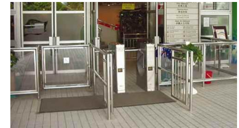
3.4.1.2h Accessible gate besides turnstiles
