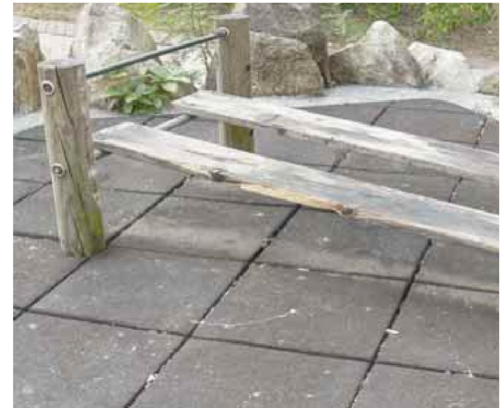
3.4.3.2j Regular maintenance to the fitness equipment is necessary
