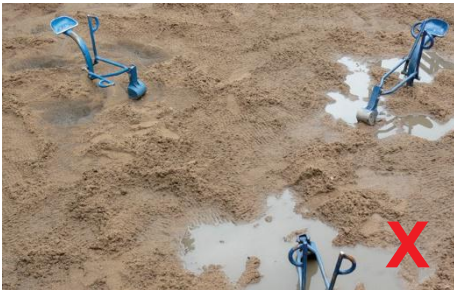
3.4.2.4m Effective drainage system at children playgrounds is essential
