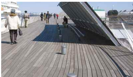
3.4.1.1c Guardrails in front of the inclined wall prevent people from walking into it and also provide shaded seating for resting
