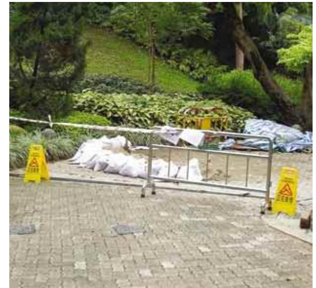
3.4.6.1e Maintenance area with guardrail and warning
