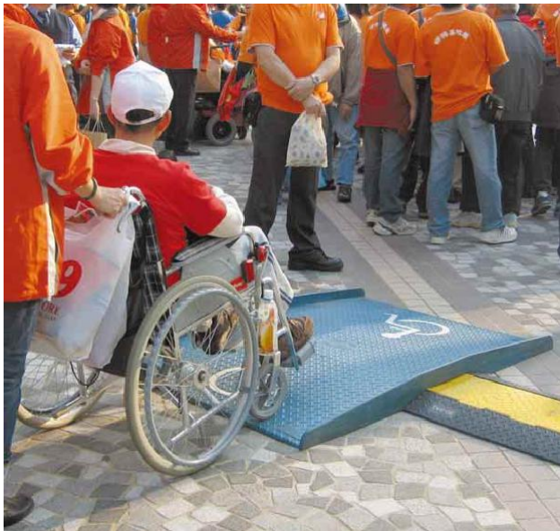
3.4.6.1c Temporary accessible ramp over covered cables running on the floor
