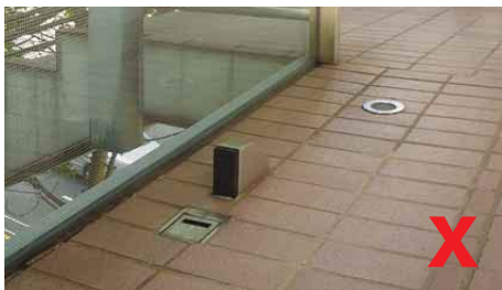
3.4.1.2d Avoid protruding gate stopper
