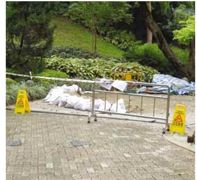
3.4.6.1e Maintenance area with guardrail and warning
