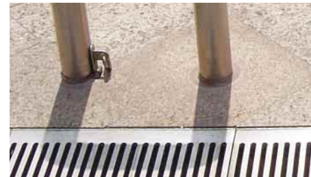
3.4.1.2f Locking device securing a guardrail post
