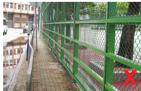
3.4.1.1d Properly supported chain-link fence (top) and deformed chain-link fence protruding onto a narrow footpath (bottom)
