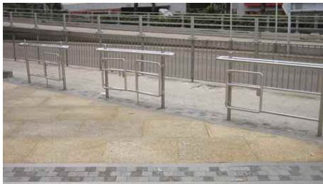
3.4.1.3a Wide opening in between guardrails
