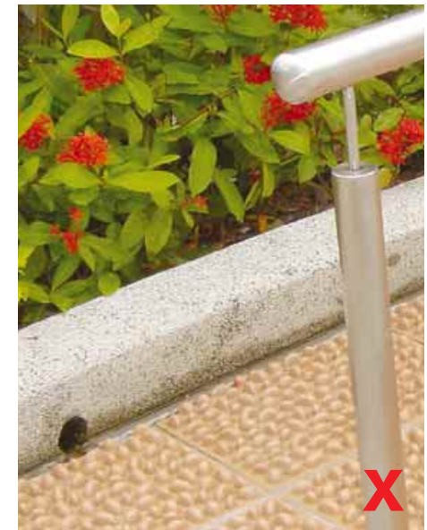
3.4.3.2c Weep-hole outlets should not be positioned directly at ground surface of outdoor exercise areas
