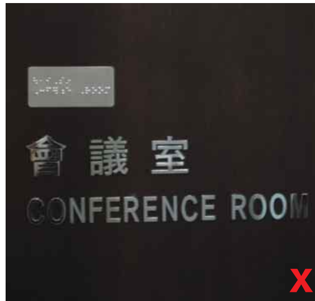
3.5.4.3a Signs made of material with a high gloss factor is difficult to read, especially if the contrast between the information and the background is low
