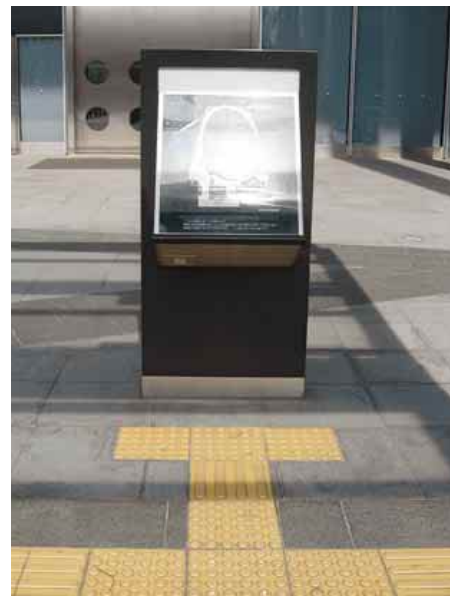
3.5.4.2a Inclined tactile directory led by tactile guide path near the building entrance
