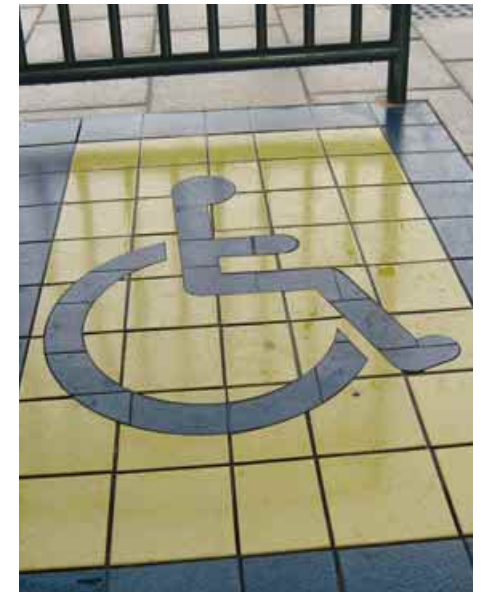
3.5.4.5a International symbol for accessibility with colour contrast to its surrounding background
