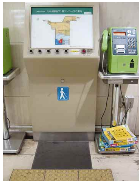
3.5.4.6a Directory with audio and Braille information, led by tactile guide path
