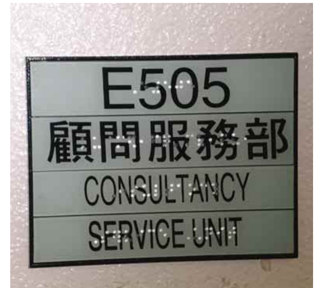
3.5.4.3b Sign in low-gloss material with Braille superimposed on top of the text
