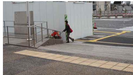
3.6.2.3a Tactile warning strips across the whole width of travel path at change in levels
