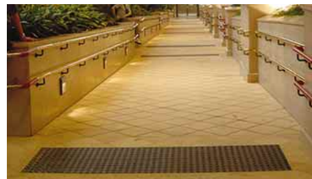
3.6.2.4a Tactiles in contrasting colour and texture to the surrounding floor finish
