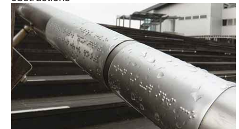
3.6.2.3n Braille information provided on handrail to facilitate way finding
