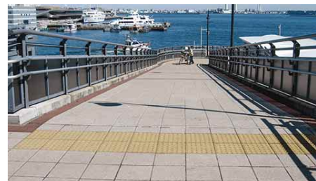
3.6.2.3d Tactile warning strips at ramp
