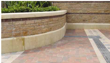
3.6.3.1b Tactiles leading to planter wall as detectable cue, users should be adequately alerted to such change in detectable surface
