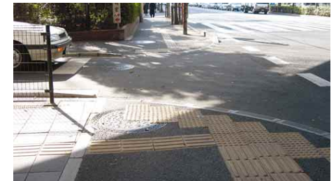
3.6.2.3e Tactiles at dropped kerb at pedestrian crossing
