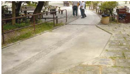
3.6.2.3g Tactile guide path along walkway with lay-by for wheelchairs
