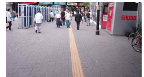
3.6.2.3f Tactile guide path on pavement
