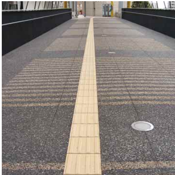
3.6.2.1a Directional tile with parallel raised bars laid along the travel direction
