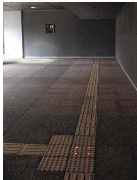
3.6.2.4c Tactiles with built-in lights inside a pedestrian subway
