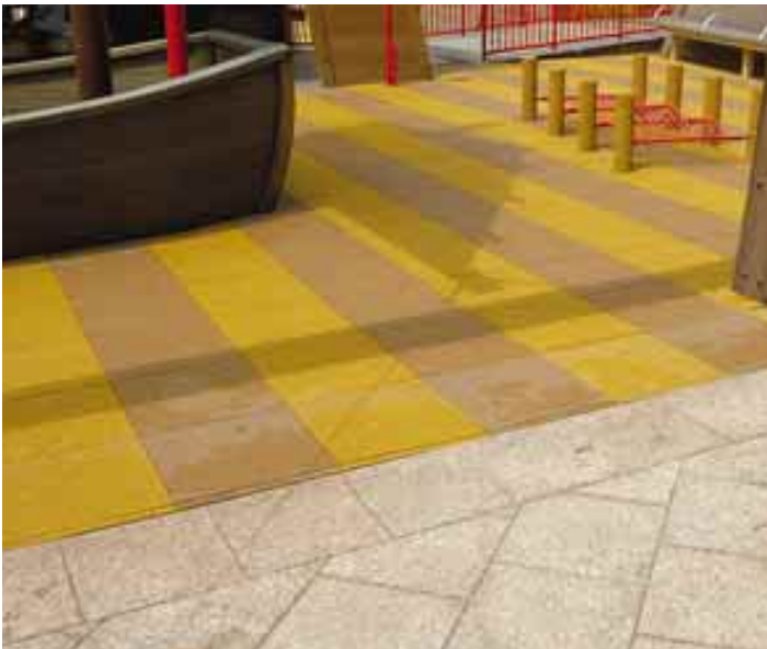
3.6.3.3a Difference in flooring materials as detectable cue to distinguish between different areas
