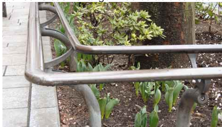
3.6.3.1c Handrails can help users to travel along a pathway
