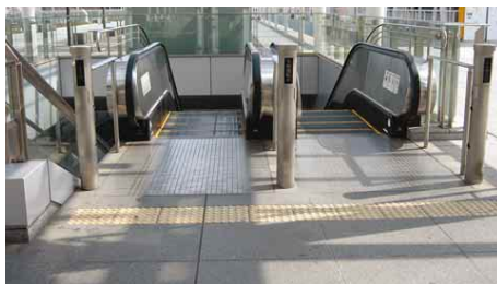
3.6.2.3h Tactile warning strips across whole width of escalators
