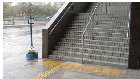
3.6.2.3b Tactile warning strips at stairways
