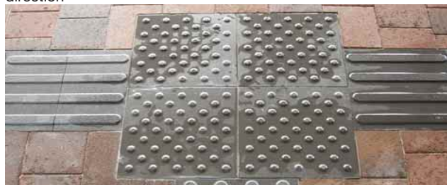
3.6.2.1c Positional tile with staggered dots positioned at junction of tactile guide path to indicate change in travel direction
