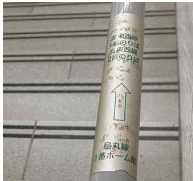
3.6.4.3a Braille on staircase handrail can identify the location as well as give information on travel directions
