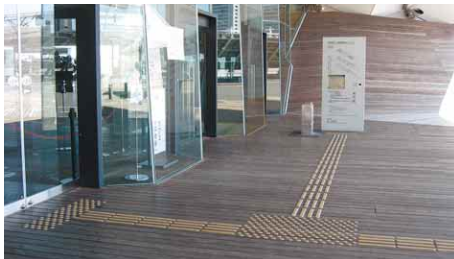
3.6.2.2a Tactile guide path at external areas leading to various areas such as main building entrance and directory
