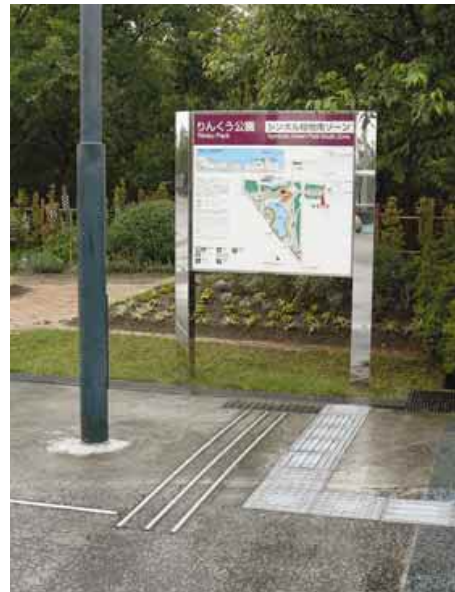
3.6.3.1d Change of detectable cues from tactile guide path to detectable strip at directory/map
