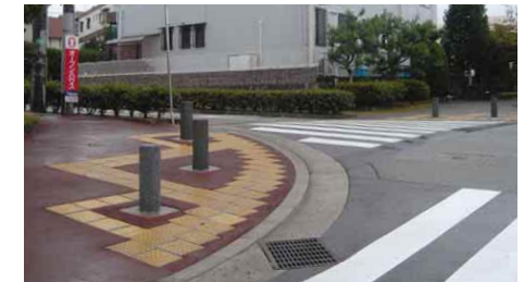
3.6.2.3m Tactiles at dropped kerb and tactiles around bollards for warning against obstructions
