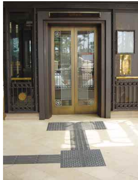
3.6.2.3i Tactiles leading to accessible lift
