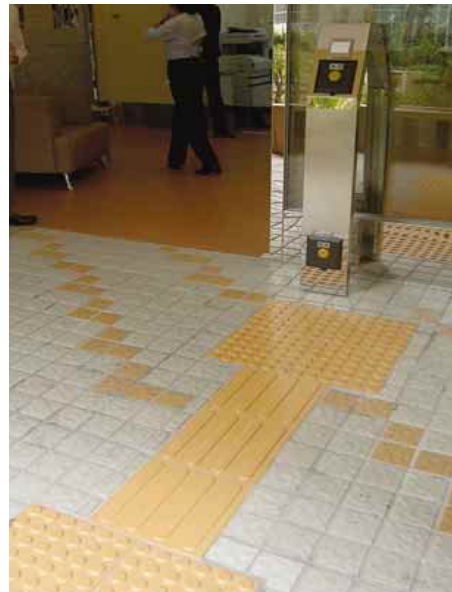
3.6.3.4a Foot or hand operable tactile door opener led by tactile guide path
