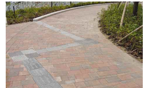
3.6.3.1a Tactiles leading to kerbs as detectable cue, users should be adequately alerted to such change in detectable surface
