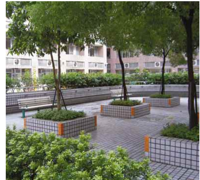
3.7.6.2b Orange colour tiles used as corner warning tiles
