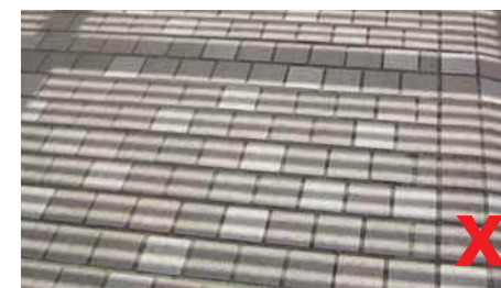
3.8.5.4c Bands of light and shade falling on an irregular floor pattern may cause a sense of dizziness to some people
