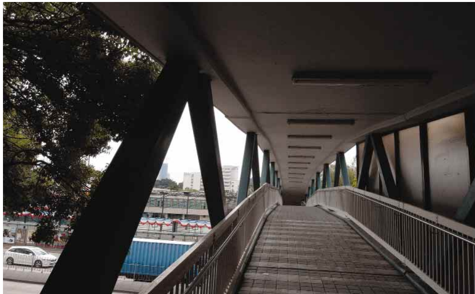
3.8.1.1a Section of walkway with uneven daylight condition
