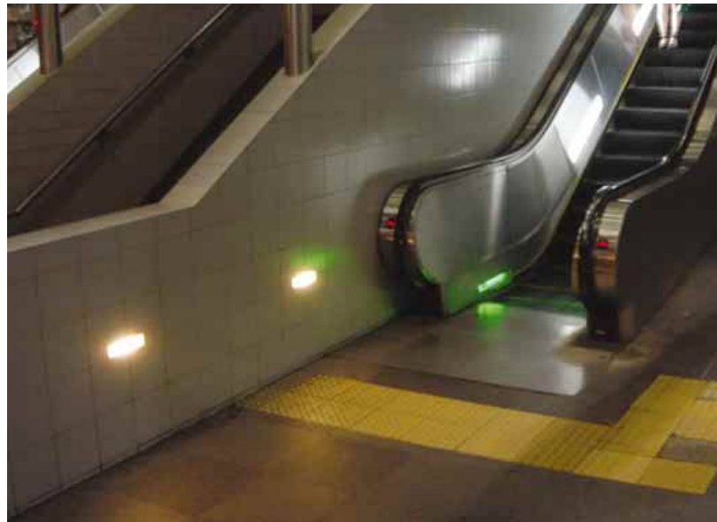
3.8.1.3c Wall-mount lighting for the area near the end of an escalator
