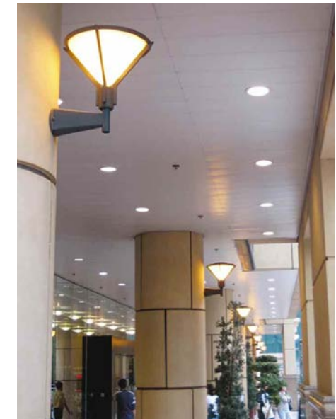
3.8.1.1c Artificial lighting to light the walkway portion with less daylight
