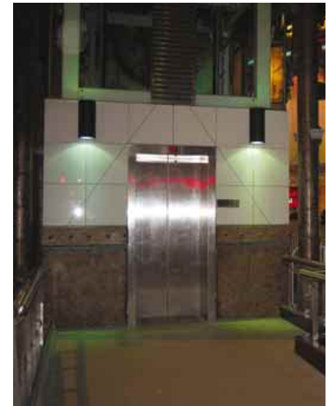
3.8.1.3d Entry to a lift for access to a footbridge with wall-mount lighting in addition to lighting for the walkway
