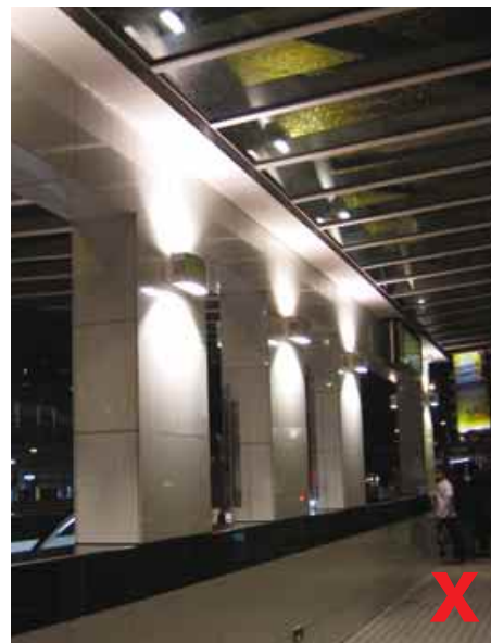
3.8.5.1b Glossy white wall surface with bright wall-mount lights creates glare
