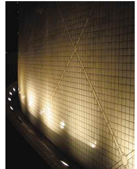
3.8.2.1c Flood light for feature wall
