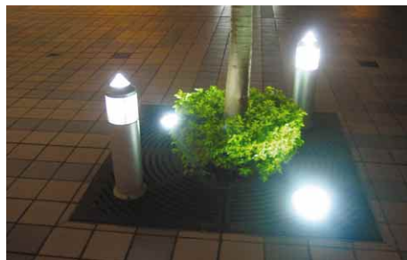
3.8.1.1d Tree pit up-light and bollard light
