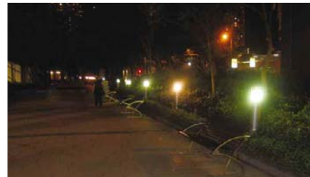
3.8.3.2a Bollard light at the planters behind the seating benches provide facial lighting but dark walking surface
