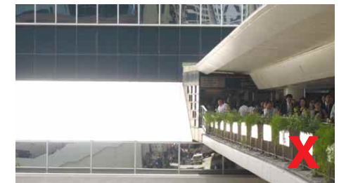
3.8.5.2a Large piece of tilted glazing beside a footbridge creates glare even after replacement with non-reflective glass
