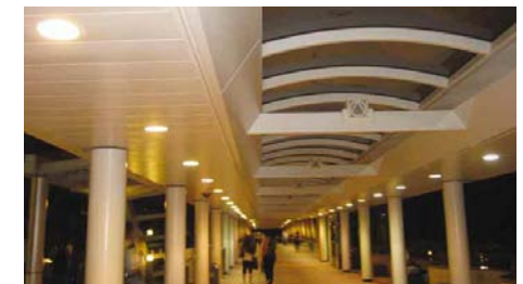
3.8.1.3b The same footbridge with double row of down lights at night
