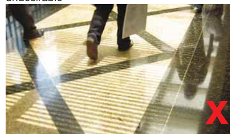
3.8.5.4b Bands of light and shade are created causing discomfort to users as they travel across the flashing bands of light and shade
