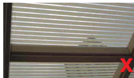
3.8.5.4a Skylight sun shading by a strip pattern perpendicular to direction of travel is undesirable
