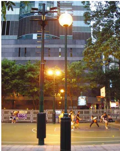
3.8.1.4a Lighting for active recreational area at night
