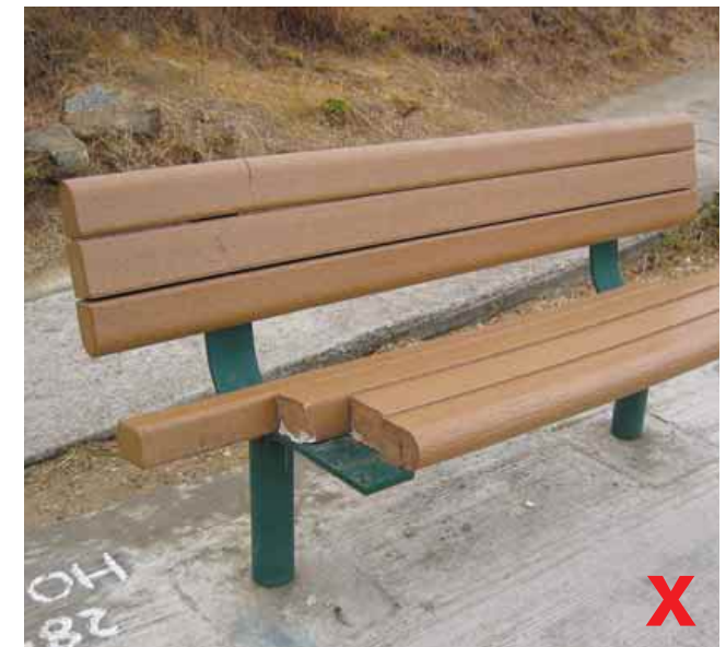
3.9.5a Poor maintenance of facilities may render them unusable or hazardous
