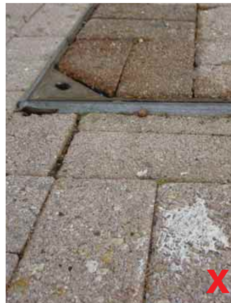
3.9.2.1c Good levelling depends on good workmanship
