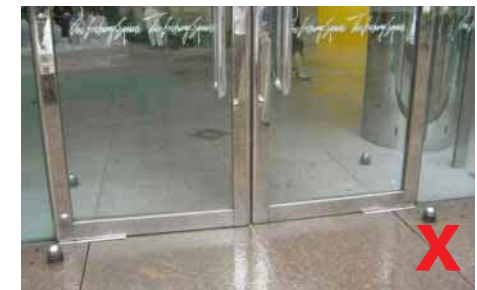
3.9.2.1d Door mat at entrance from outdoor to indoor can help prevent slips and falls
