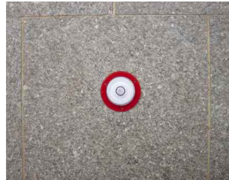
ii) Check levelling of ground surface to be tested
