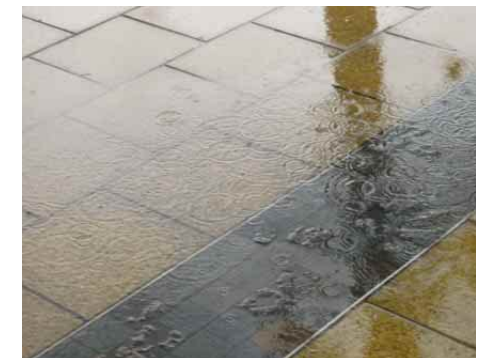
ix) Repeat the test under wet condition during rainfall
