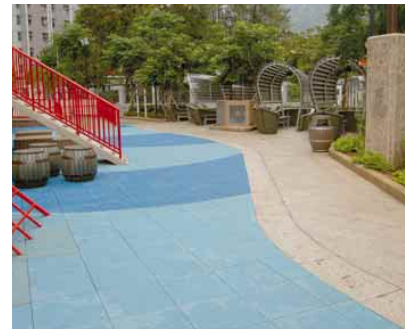
4.1e Use of different flooring materials to demarcate main access paths from the other functional areas
