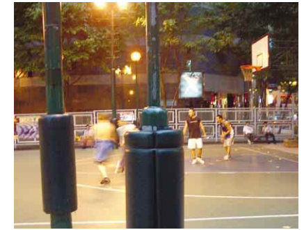
4.4ff Lamp poles near basketball courts wrapped with protective cushion
