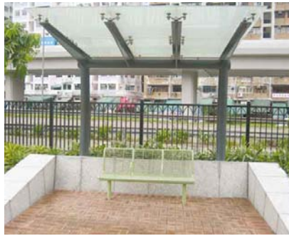
4.4a Covered seating bench with adjoining wheelchair space recessed from the walkway
