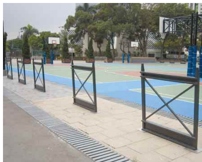
4.4g Wide clearance provided in between barriers that demarcate areas for different activities
