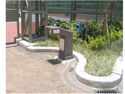
4.4w Drinking fountain with leg room for wheelchair and placed in a recess
