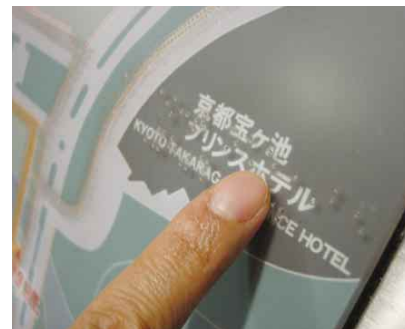
4.4s Tactile map with Braille description mounted at an angle for easy reading and touching
