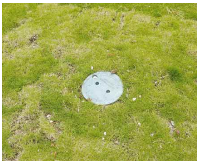
4.4r Pop-up sprinklers flush with the finished level of an accessible lawn
