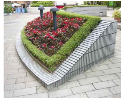
4.4p Inclined planter box for better visual contact and close reach for viewers of different heights
