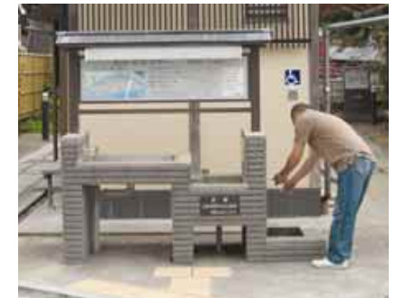
4.4q Provision of sinks and taps at different heights to cater to a wide range of users
