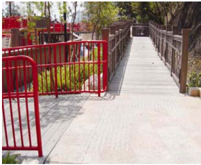
4.4j Ramps with tactile warning strips and handrails fixed at suitable height on both sides
