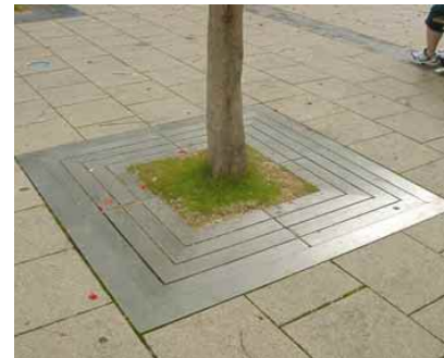
4.4y Tree pit cover with narrow slots installed levelled with the surrounding ground surface
