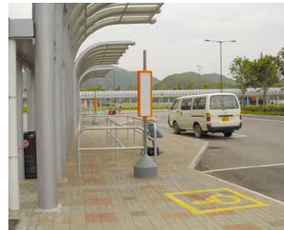
4.5p Signage at public transport facility identifying the designated accessible pick up/drop off point
