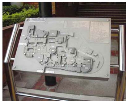
4.5g Three-dimensional tactile directory helping users with different abilities to formulate an overall picture of their surroundings
