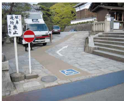
4.5r Designated accessible path for wheelchair users identified by international symbol for accessibility
