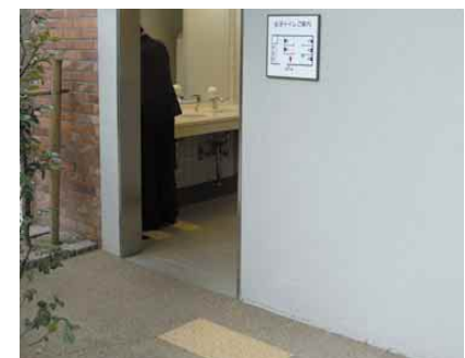
4.5t Tactile warning strips leading to a tactile directory for sanitary facilities
