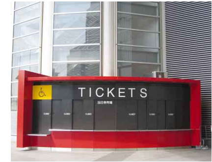
4.5f Large signage with international symbol of accessibility in contrasting colours indicating an accessible service counter
