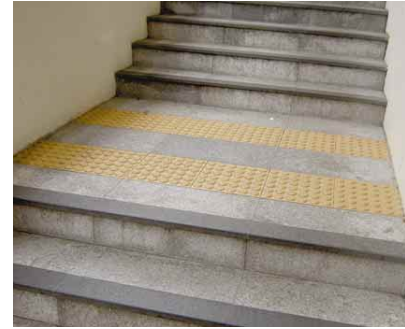
4.6b Tactile warning strips at staircase landing
