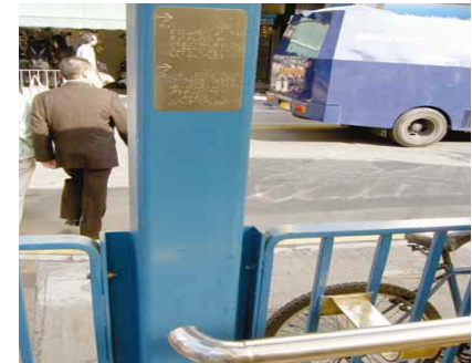
4.6q Braille information on a guard rail post to indicate travel direction
