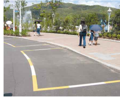
4.6k Pick-up/drop-off point with dropped kerb and tactile guide path leading to an accessible entrance
