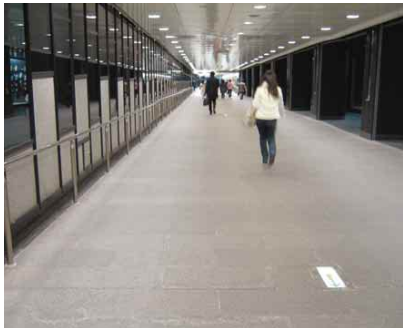
4.6n Continuous handrails provided along the travel path to facilitate access
