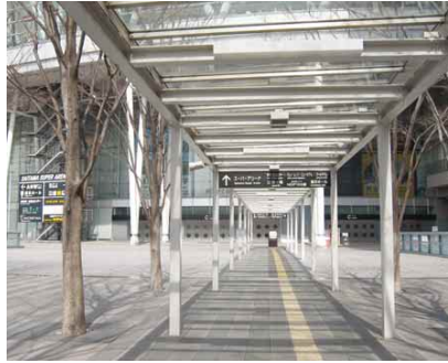
4.6a Tactile guide path along an external covered walkway to facilitate access
