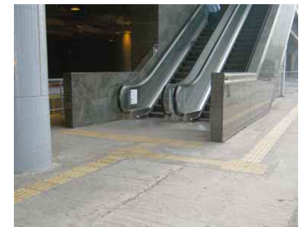
4.6i Tactile guide path leading to transport facilities and connection to other destinations
