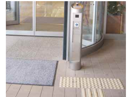
4.6f Tactile guide path leading to automatic door opener with high/low control buttons at the building entrance
