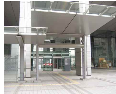
4.6e Tactile guide path leading to main building entrance
