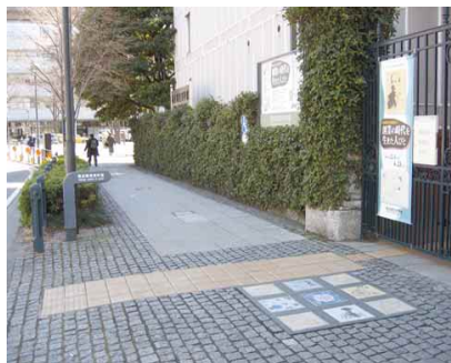
4.6g Different paving materials identifying different areas and tactile warning strips provided across the width of the pavement to alert users of an entrance
