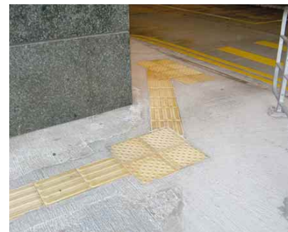
4.6h Tactile guide path leading to transport facilities
