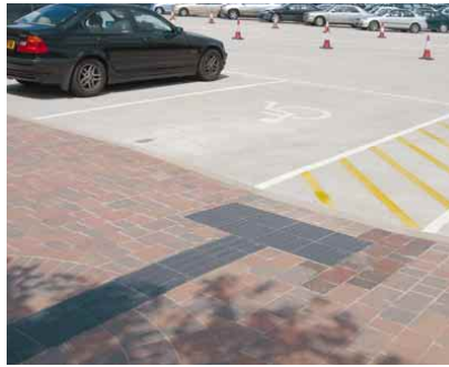
4.7dd Tactile guide path leading to an accessible car park accented by the distinct contrast between the black tactiles and the red paving
