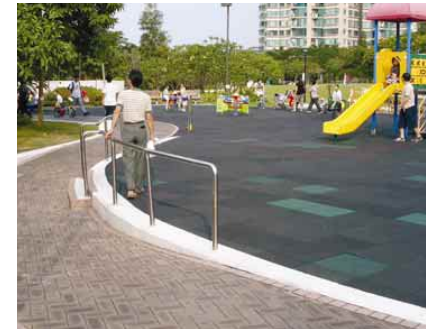
4.7ff Black rubber mats forming a backdrop for the colourful play equipment; the contrasting flooring colours and textures effectively demarcate the play area from the access paths
