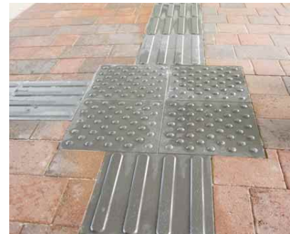
4.7y Black tactile guide path forms a good contrast with the surrounding reddish brown paving
