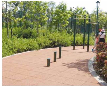
4.7d Use of red floor finishing to distinguish the access area from the soft landscaping areas; the edge junction is emphasized by white borders for further visual contrast
