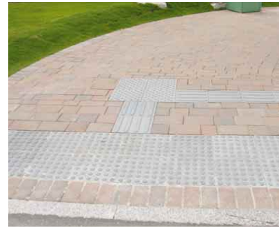
4.7ee Contrast created by black tactile guide path on red paving access path
