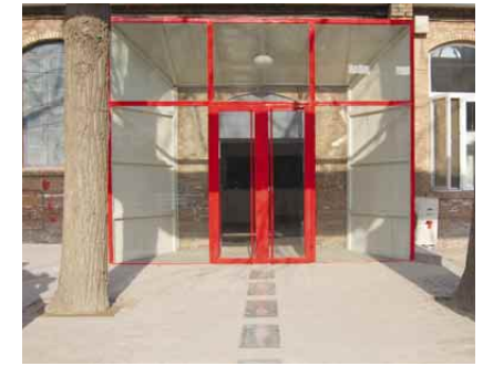
4.7c Entrance door frame in bright red forms a strong contrast with, and stands out from, the surrounding materials
