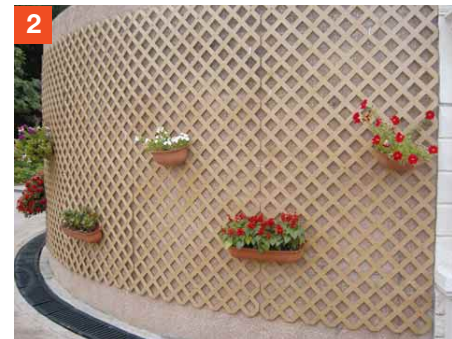
A1.6.1h Trellises with hanging baskets for vertical greening or displaying artwork created by the boarders
