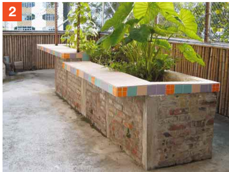
A1.4.1i Potting table designed with leg room and drop height for different users
