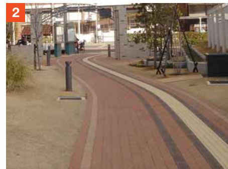
A1.5.1i Tactile cues to improve sense of orientation for the visually impaired
