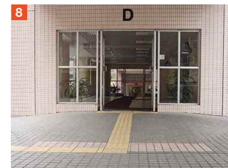
A1.3.1q Levelled entryway with tactile path
