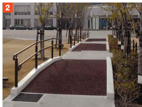
A1.3.1j Rubberised exercise ramp can cushion falls and is also firm enough for wheelchairs
