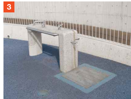
A1.4.1j Washing basin with drop height to suit a wide range of users
