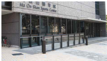
A2.3.4c Tactile warning strips provided at top and bottom of access ramp to Sports Centre
