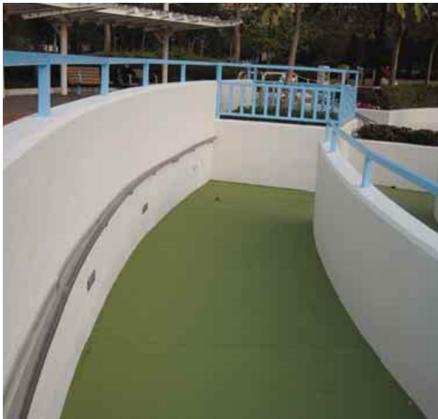
A2.6.3a Handrails at ramp
