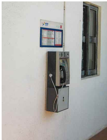
A2.7.1a Pay phone mounted at low level outside the Park Office
