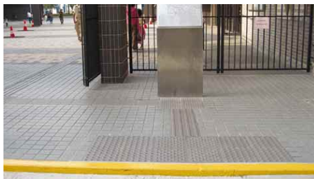
A2.4.1b Entrance to the Public Library and Sports Centre with tactile map and tactile guide path
