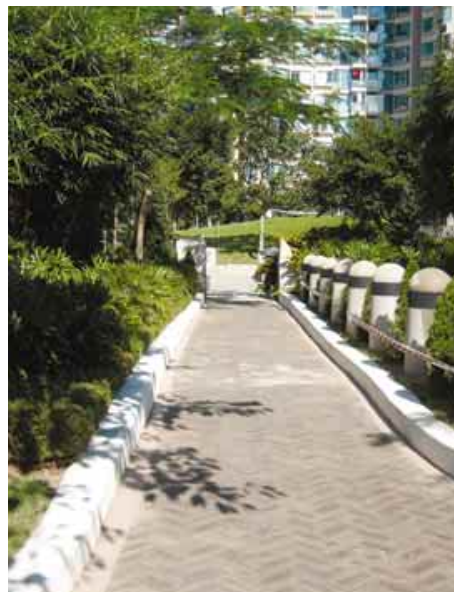
A2.3.4e Detectable kerb along access route with colour contrast to adjacent floor finish
