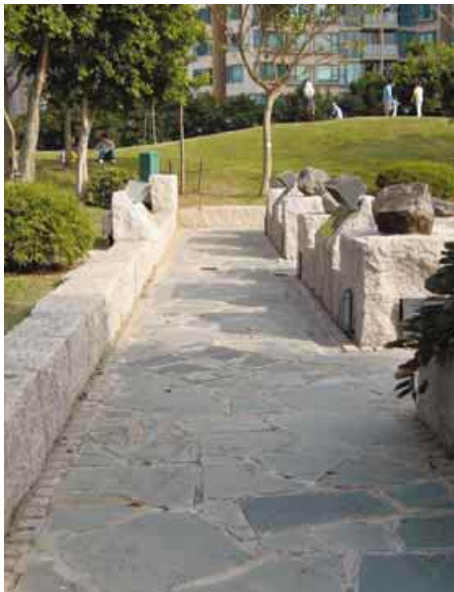
A2.3.5a Natural stone paving at Mining History Display Area
