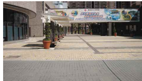
A2.3.5b Different ground surface materials for the plaza and the vehicular pathway
