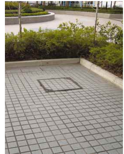
A2.3.6c Manhole covers levelled with the surrounding floor surface. Junction between different floor finishes are also levelled
