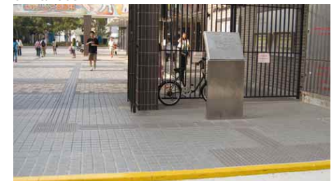
A2.3.4b Tactile guide path provided from site boundary to tactile map and leading to the building entrances
