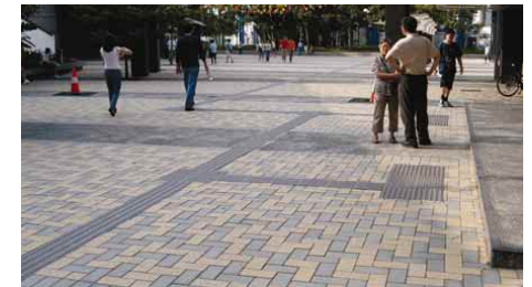
A2.3.4a Clear access route with tactile guide path leading to the Library and Sports Centre entrances
