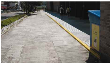
A2.3.3b Yellow warning strip at pavement kerb outside Library entrance
