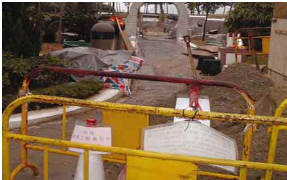
A2.12.1a Repair works cordoned off with temporary barriers
