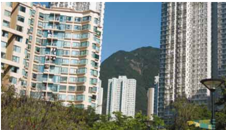
A2.4.2a The nearby tall residential buildings form a reference point for orientation
