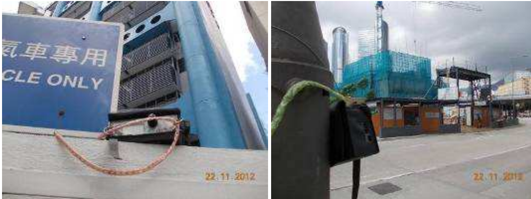
Photo 5. Monitoring of Total Suspended Particulate (TSP)
