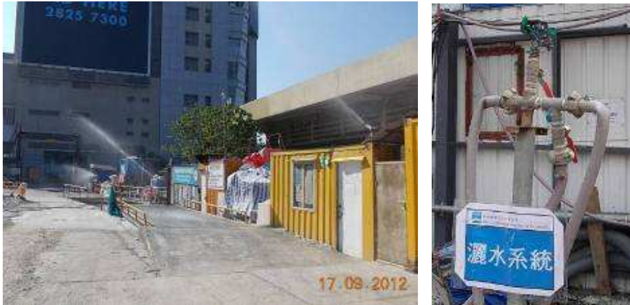
Photo 1. Provision of Spray Sprinkler System at main access for dust suspension
