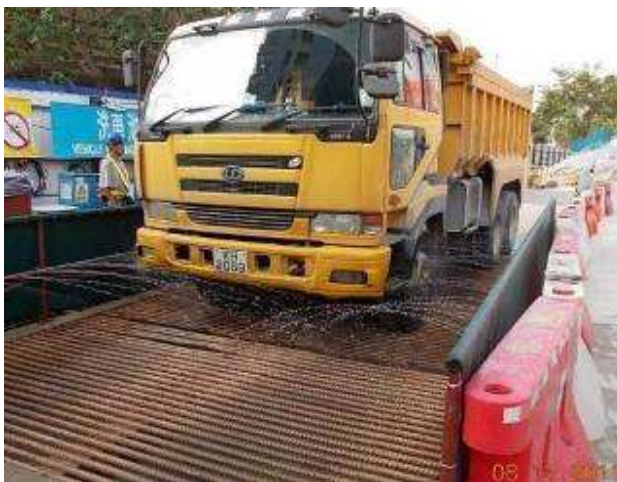
Photo7. Automatic wheel washing facility was provided on site
