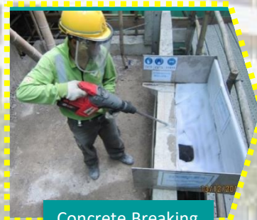
Concrete Breaking
