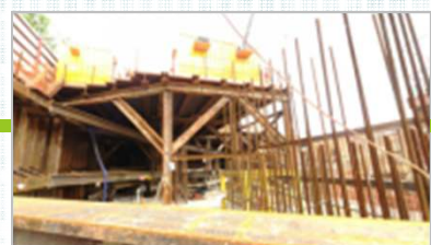
挖掘與側向承托興建
