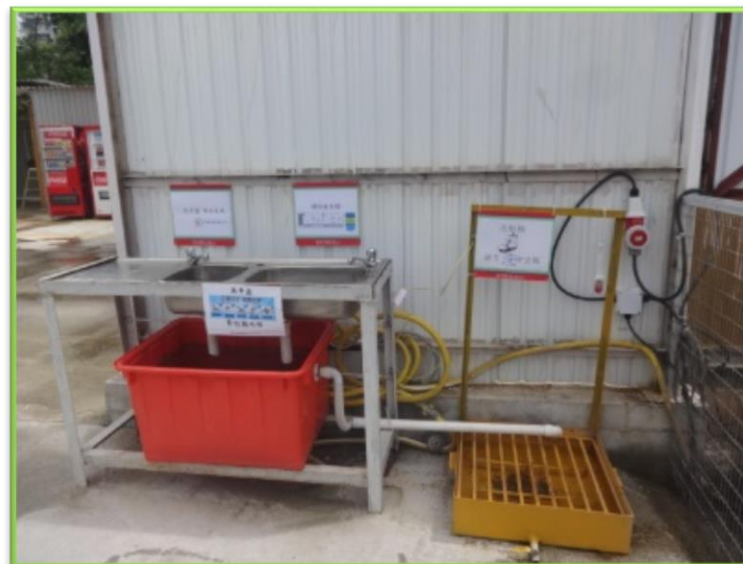
Using recycle water for shoes cleaning bath
