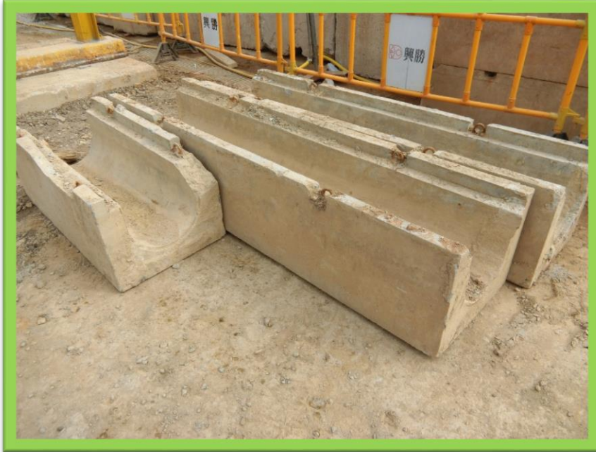
Pre-cast UU channel to reduce wastage
