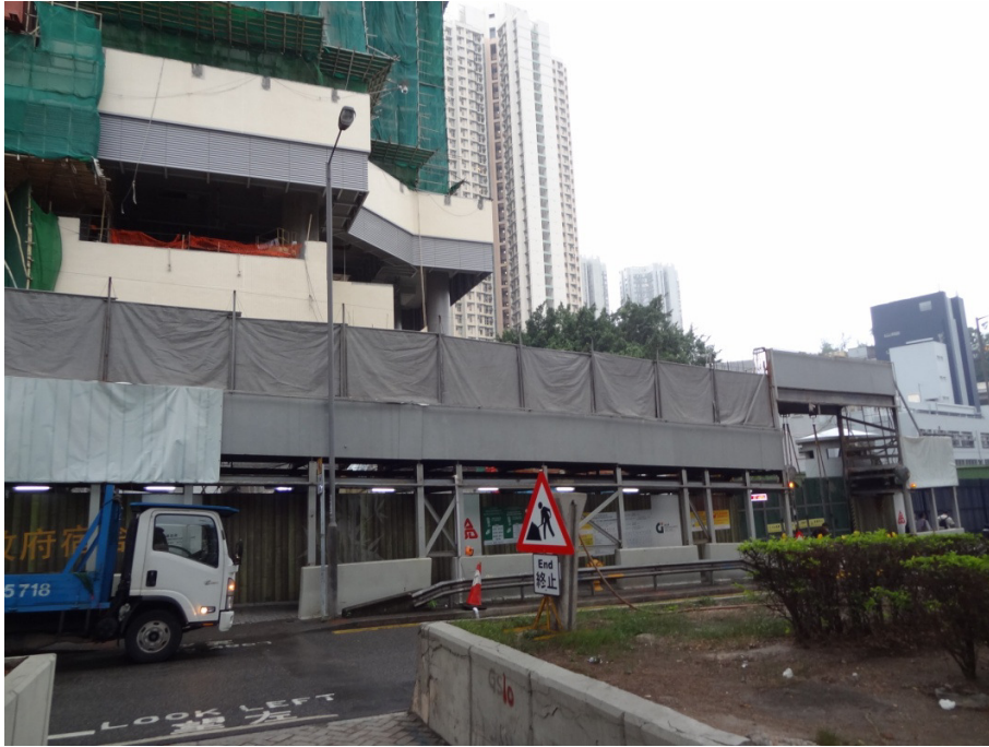
Erection of additional noise screening tarpaulin on hoarding
