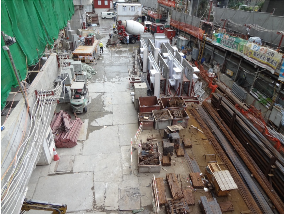
Adopt hard-paving construction - Reduce muddy water and fugitive dust
