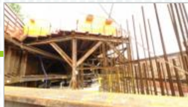
挖掘與側向承托興建
