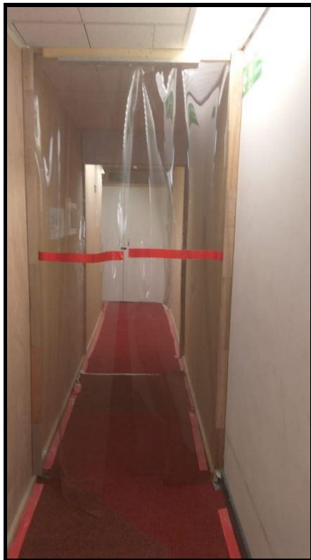
Dust Screen at long corridor leading to Exist
