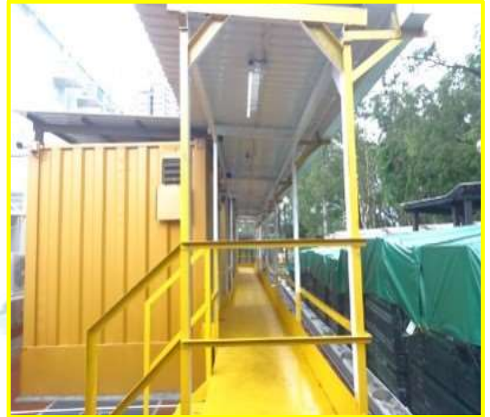
Motion sensors for lighting system
