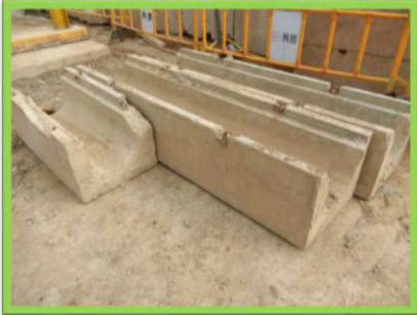
Pre-cast UU channel to reduce wastage
