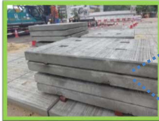
Pre-cast hard paving to reduce the dust emission
