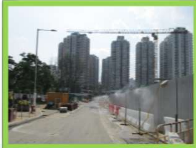
Water Spraying System for dust suppression
