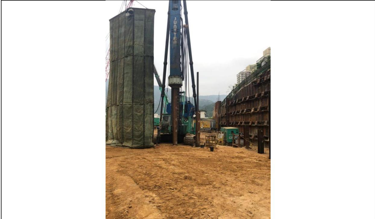
Hoisting of noise barrier during piling
