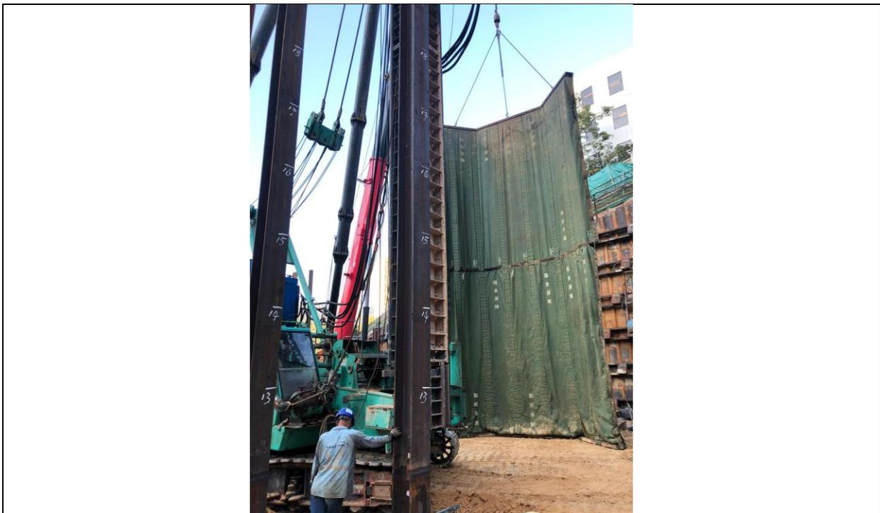
Hoisting of noise barrier during piling
