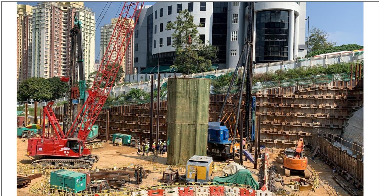
Hoisting of noise barrier during piling
