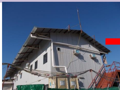
Rainwater harvesting system at site office for cleaning purpose
