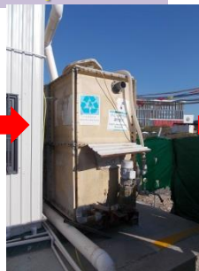
Rainwater harvesting system at site office for cleaning purpose
