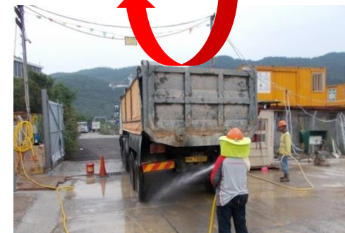
Reuse treated water for wheel washing
