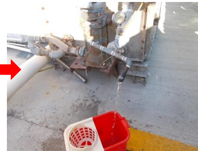
Rainwater harvesting system at site office for cleaning purpose
