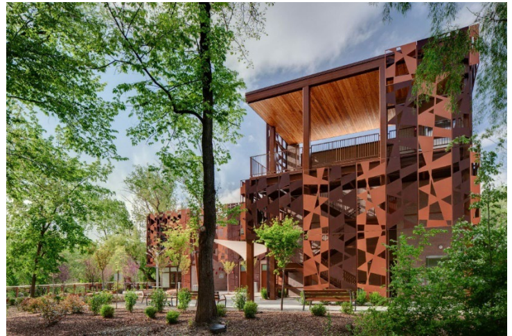
The Tracy Aviary's new LEED Gold Visitors Center meets the requirements of LEED's Reducing Bird Collisions credit, using an array of high- and low-tech solutions, including decals and a dramatic screen.
