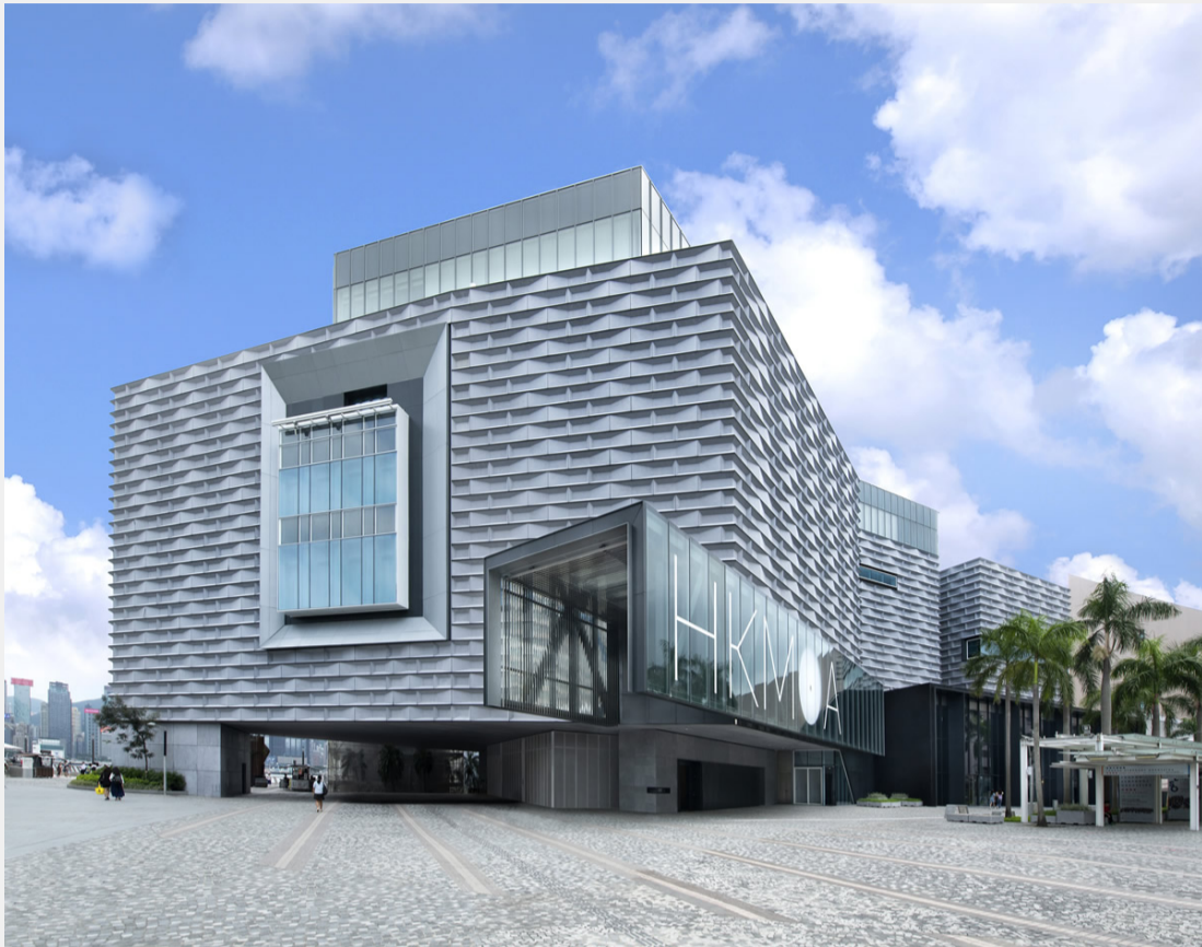
New building canopy
