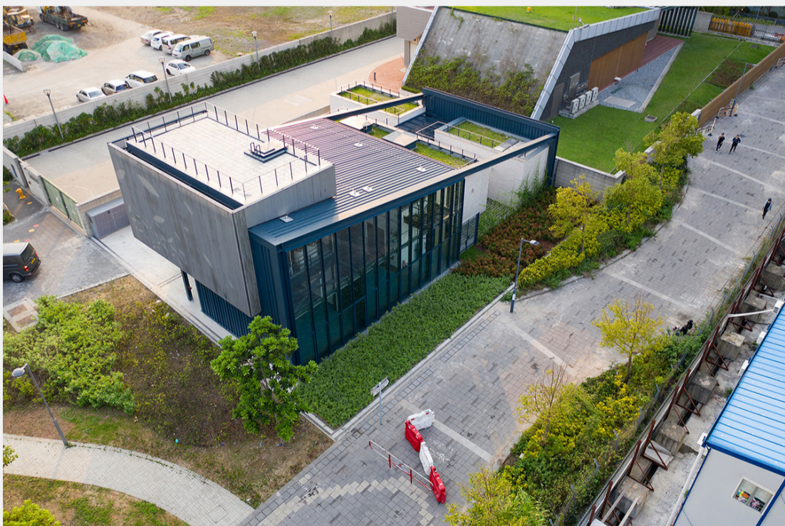
Aerial view of the new RCP
