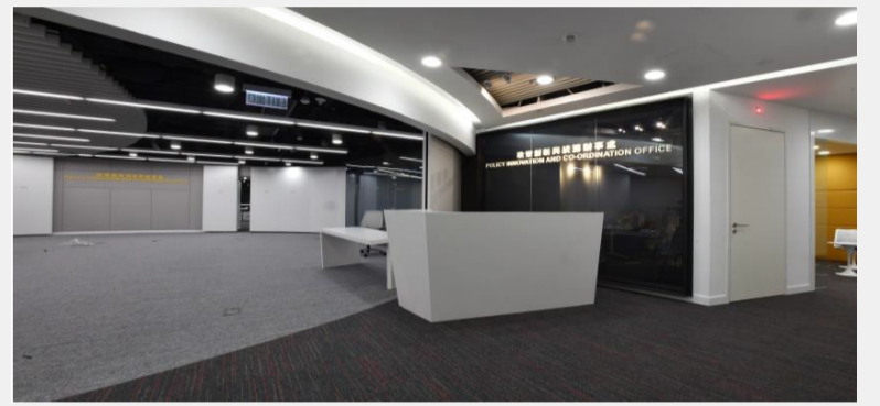
Use of energy efficient LED lighting in the reception area is improved by motion sensors
