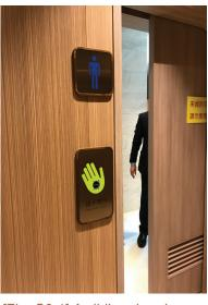
[Fig. C3.1] A sliding door is fitted with hands-free operator that helps the elderly to open/ close the door easily.
