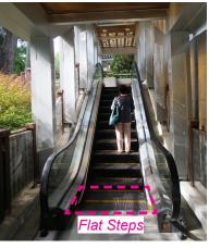
[Fig. B7.1] Flat step is a step that is level with the landing prior to rising or descending along the incline.
