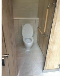
[Fig. E2.2] Grab bars should be provided on both sides of the water closet.
