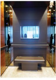
[Fig. B8.1] Provision of seat in lift car for frail passengers should be considered for buildings frequently visited by the elderly.
