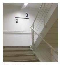
[Fig. B5.3] Appropriate sign that identifies floor level should be provided at landing.
