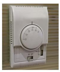
[Fig. C5.1] A thermostat with an user friendly dial allows easy adjustment of room temperature
