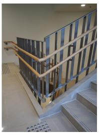
[Fig.D2.1] Dual-level handrails should be considered to cater for people with different physical conditions.
