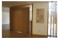
[Fig. B4.2] Rounded or splayed corner at right angle turn can minimize risk of injury.
