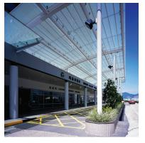
[Fig. B2.1] A large canopy at passenger drop-off and pickup point for weather protection.
