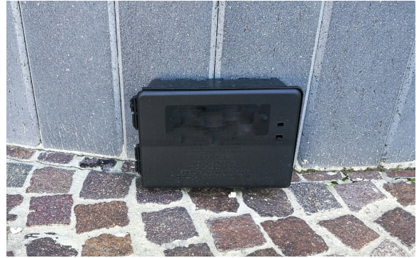
▲ Example of Smart Pest Control System
