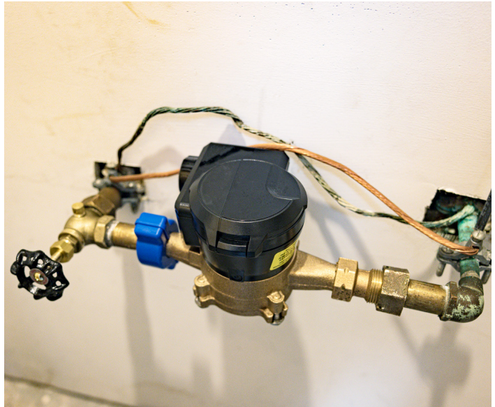
▲ Installation of Smart Water Meter
