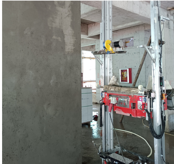
Automated Wall Plastering Machine
