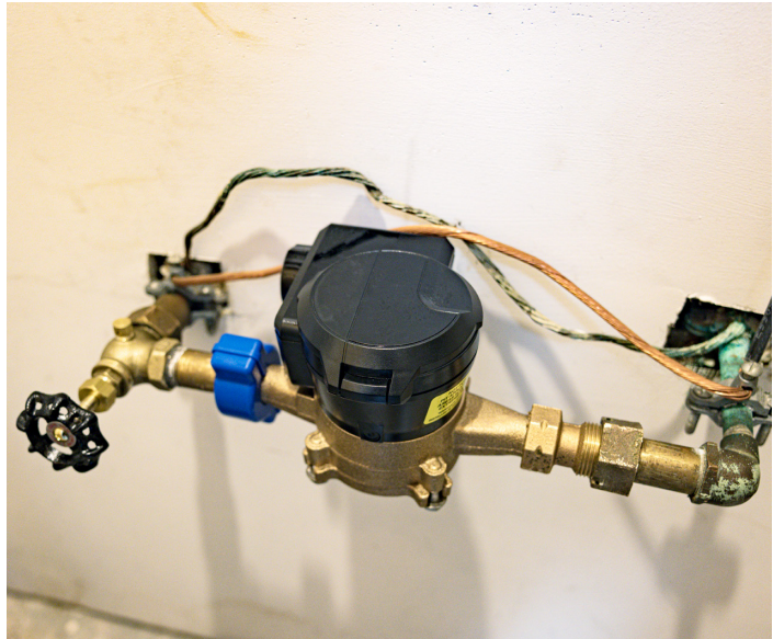
▲ Installation of Smart Water Meter
