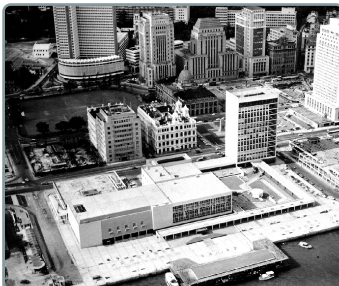
Hong Kong City Hall, 1950s
